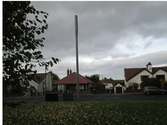
Photo looking north across Wilthorpe Road.
