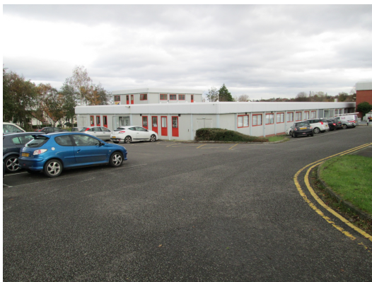
Photo looking north east to adjacent existing building.
