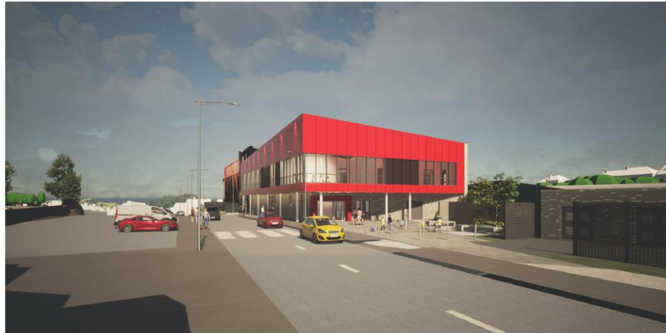
View from Station Entrance
