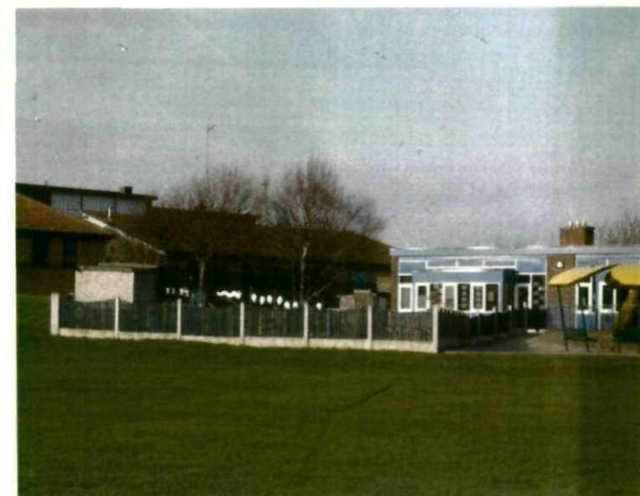
5. Rear of Classrooms
