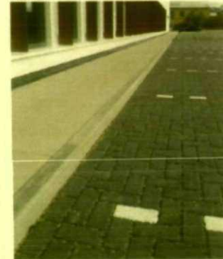
Concrete Road Kerb
