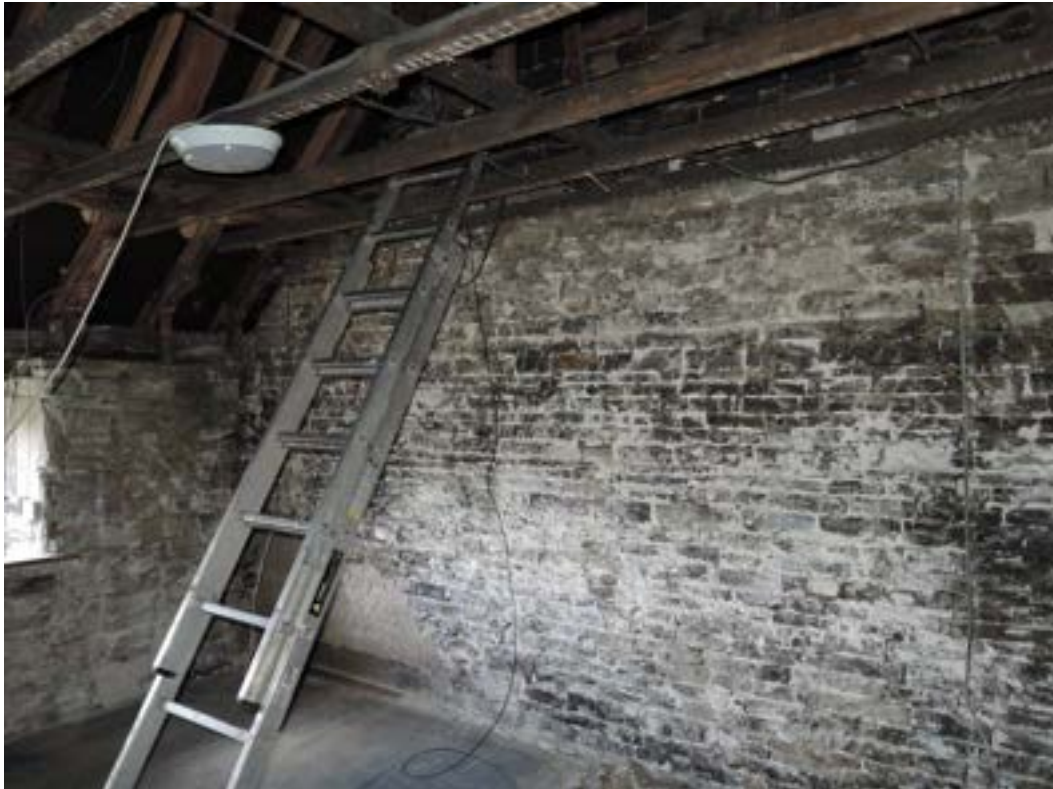
Inside southwest gable
