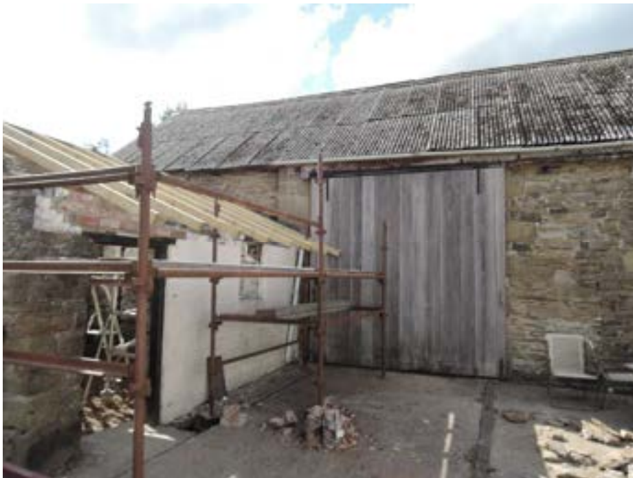
Large barn at south end of yard
