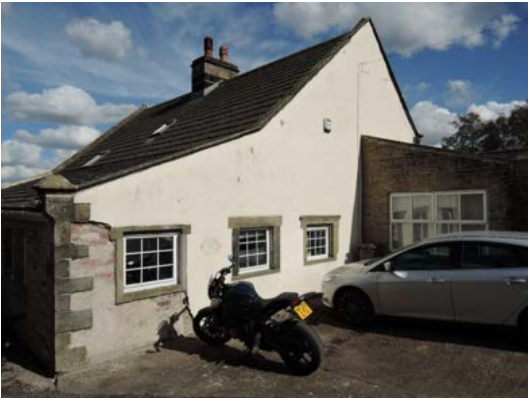
Southwest gable. Brickwork revealed under render to extension
