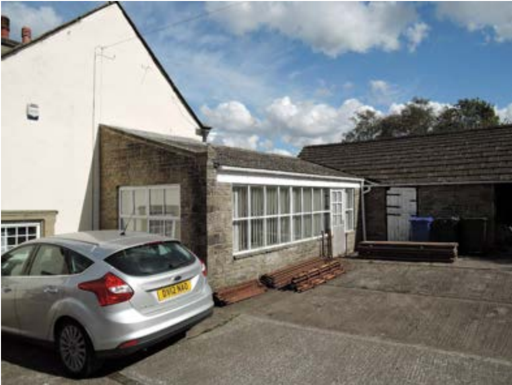
Single storey extension in yard, to be replaced.
