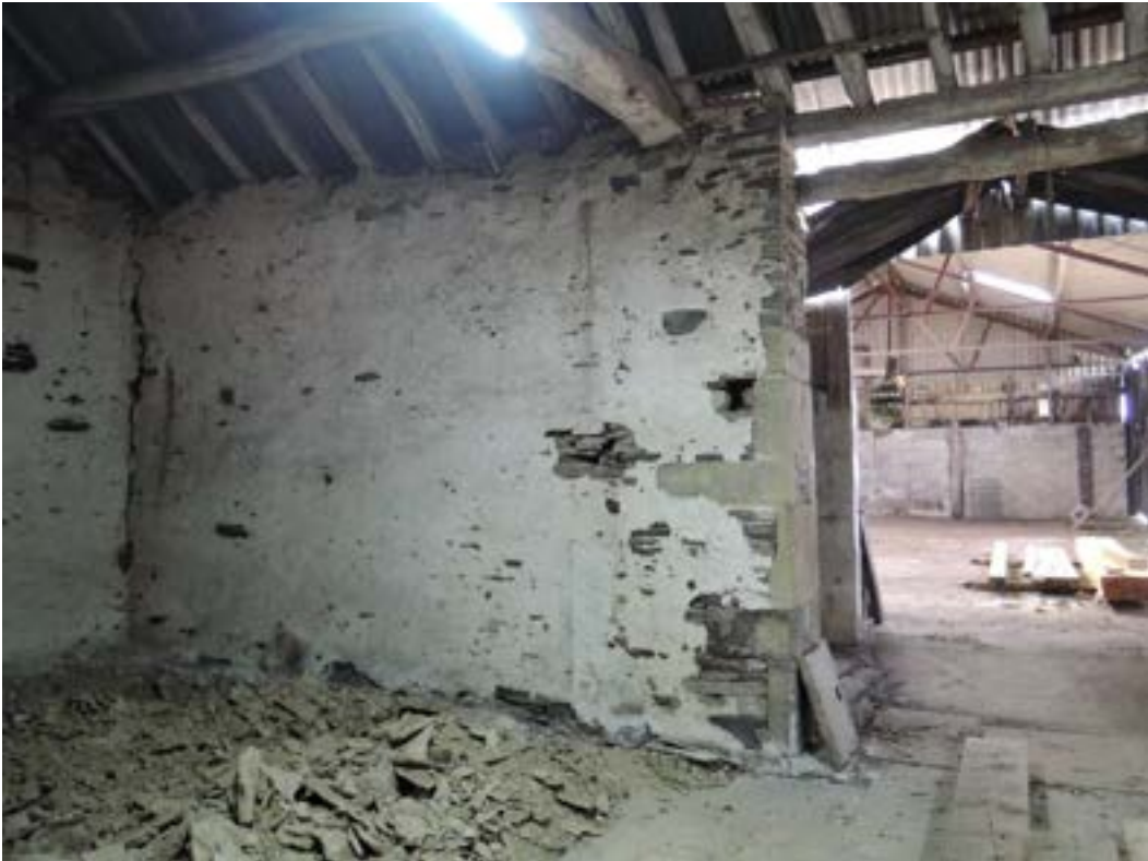
Flank wall (gable on left) entrance to barn to be demolished.
