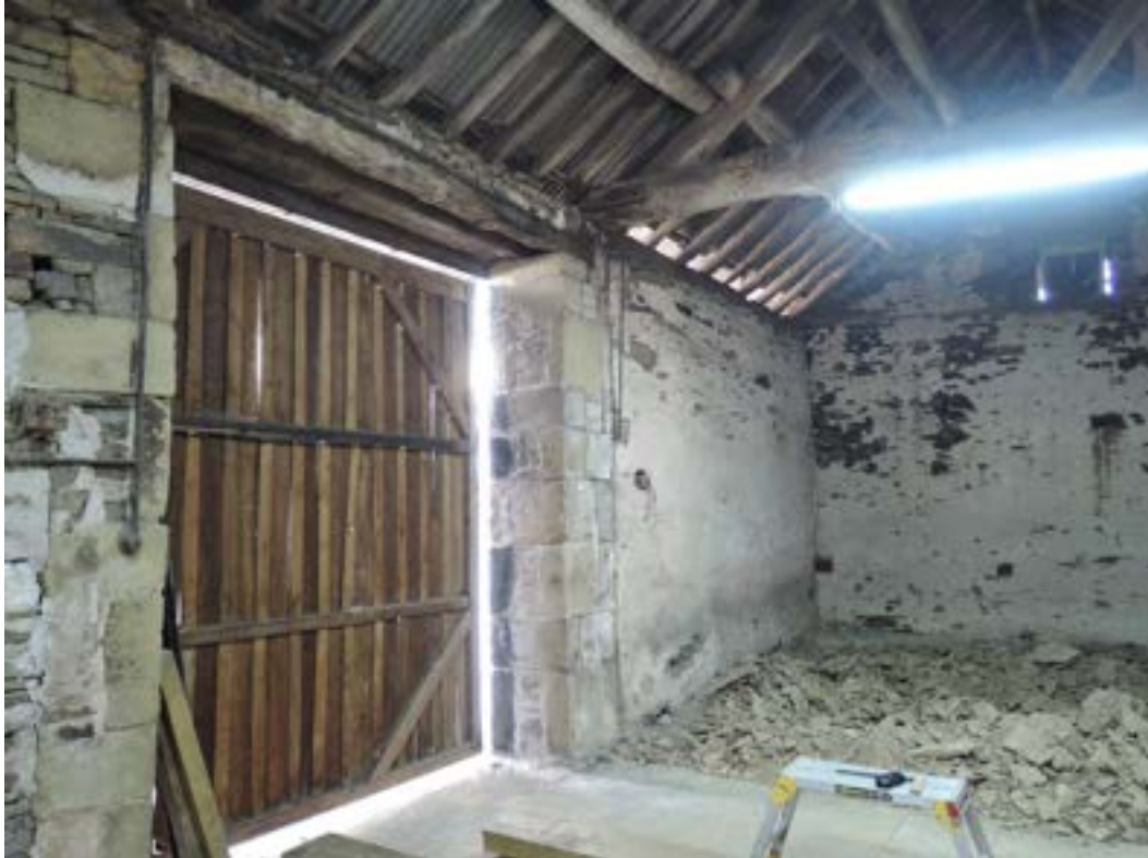
Large barn southeast corner
