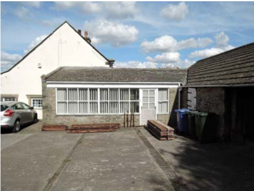
Single storey extension in yard. Cottage gable in good order
