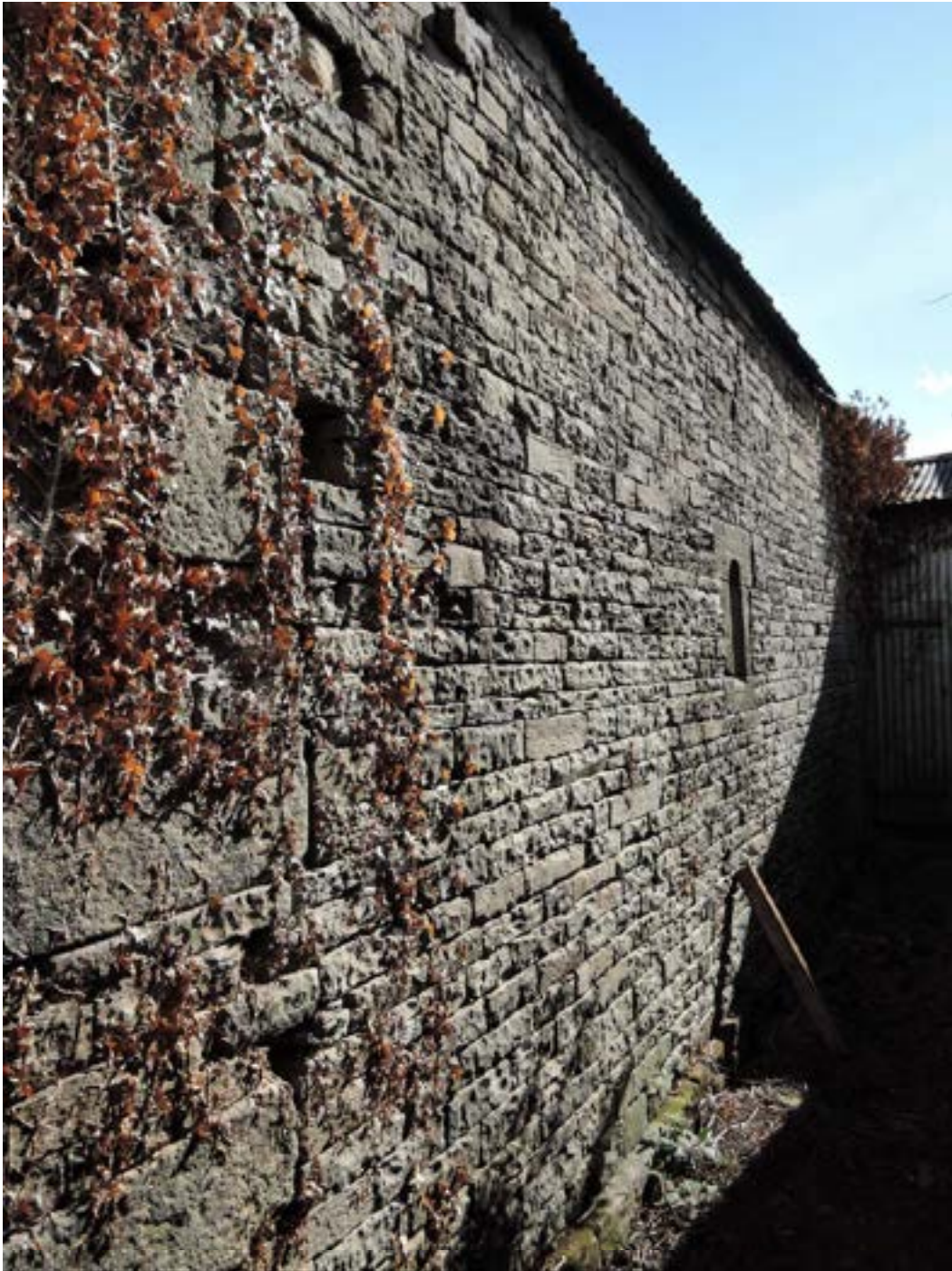
Large barn back wall looking south
