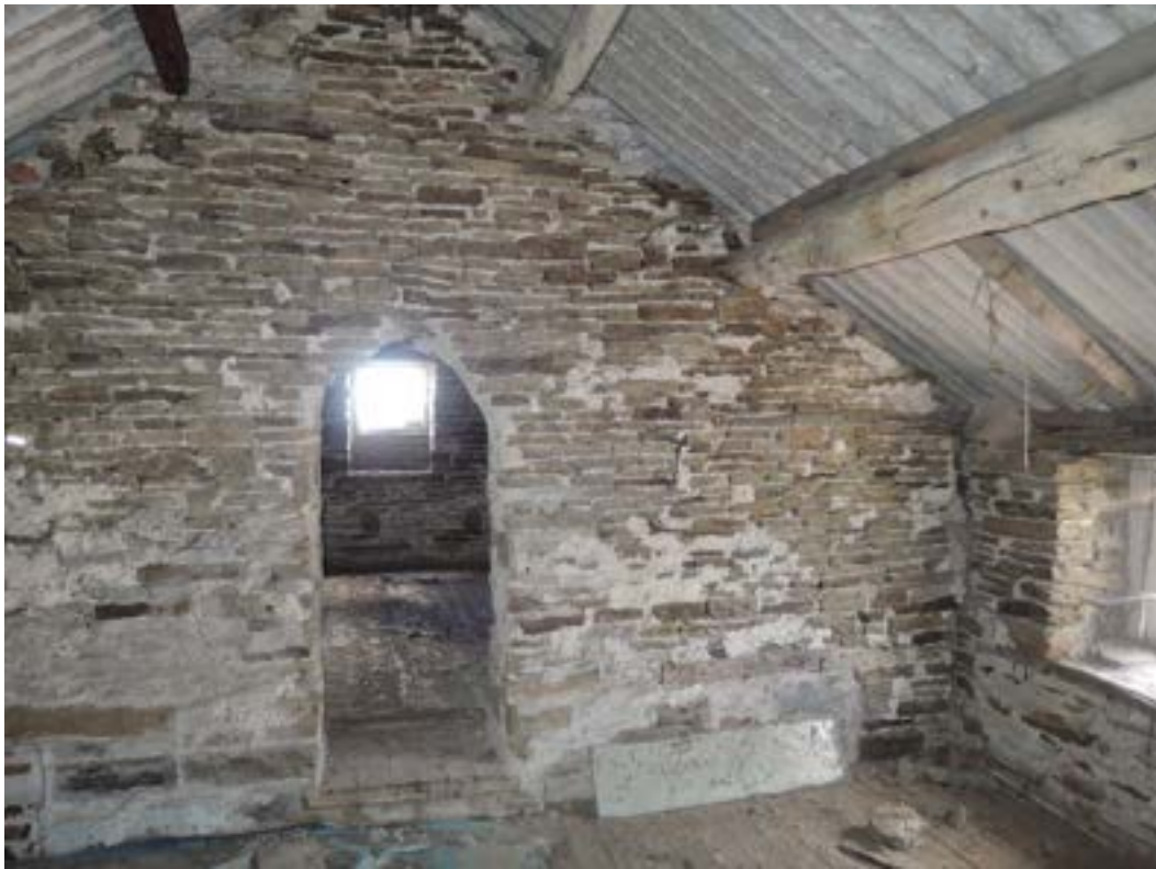
1st floor small barn intermediate wall
