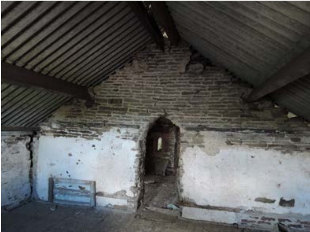
1st floor intermediate wall small barn (same wall as previous pic)
