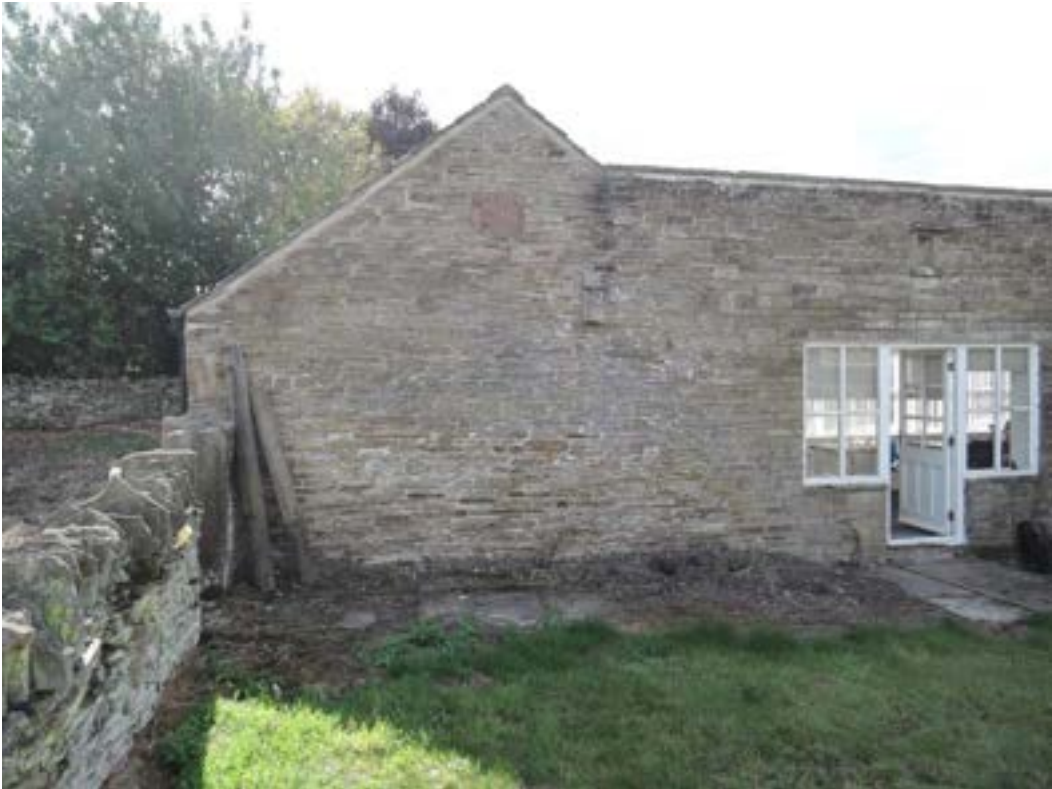
Gable to shed/garage in good order
