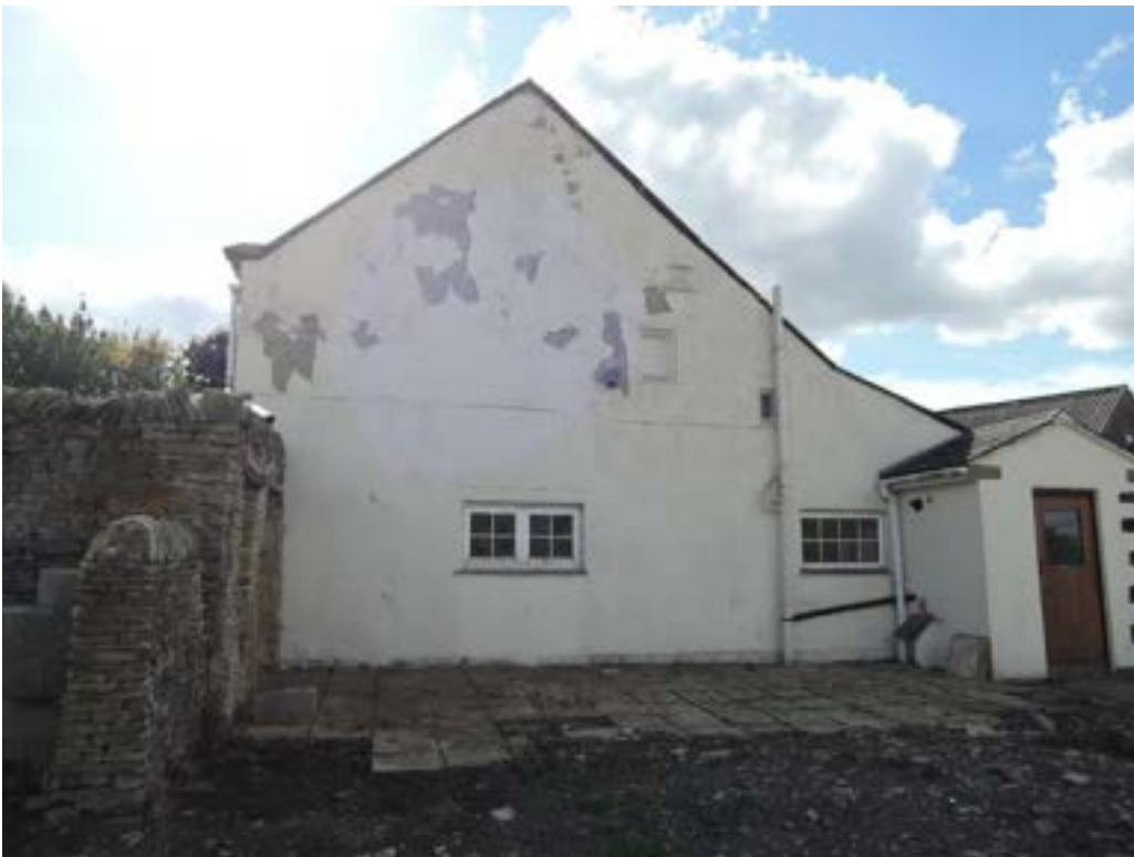
Northeast gable. Tired and peeling paint/render but no major cracks or bulging apparent.
