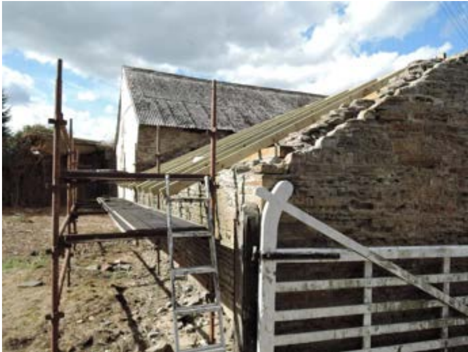
Low level shed under repair receiving new roof. Large barn in background.
