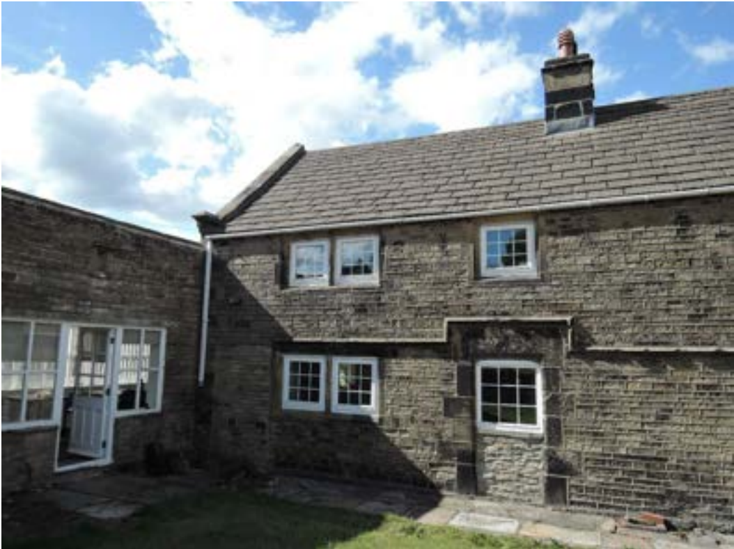
Left end of garden elevation. Extension on left to be replaced
