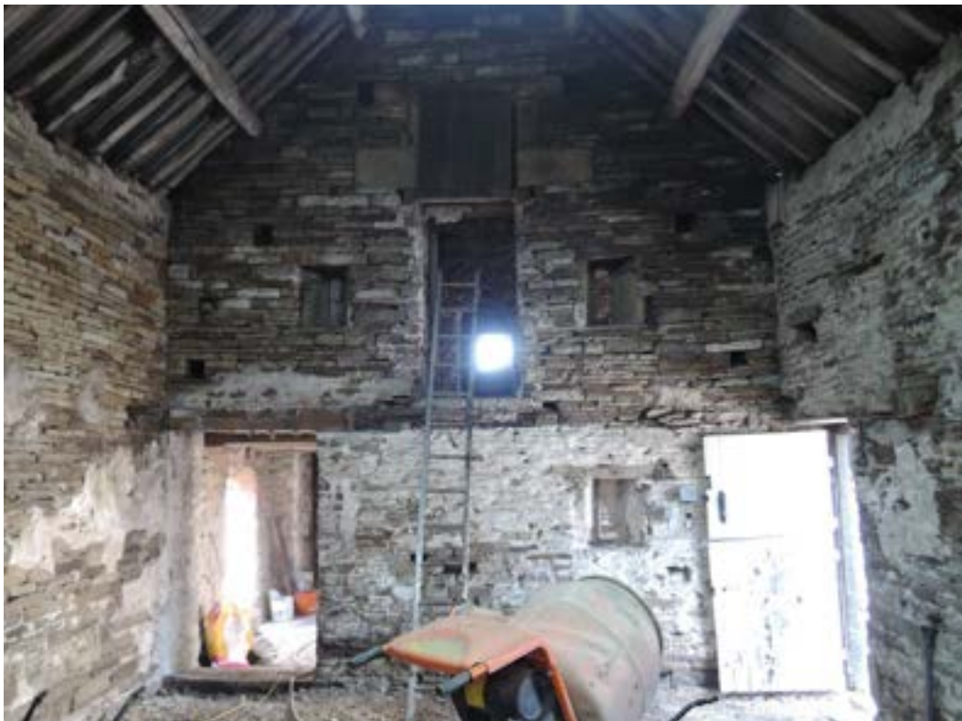
Party wall to large/small barn looking north.
