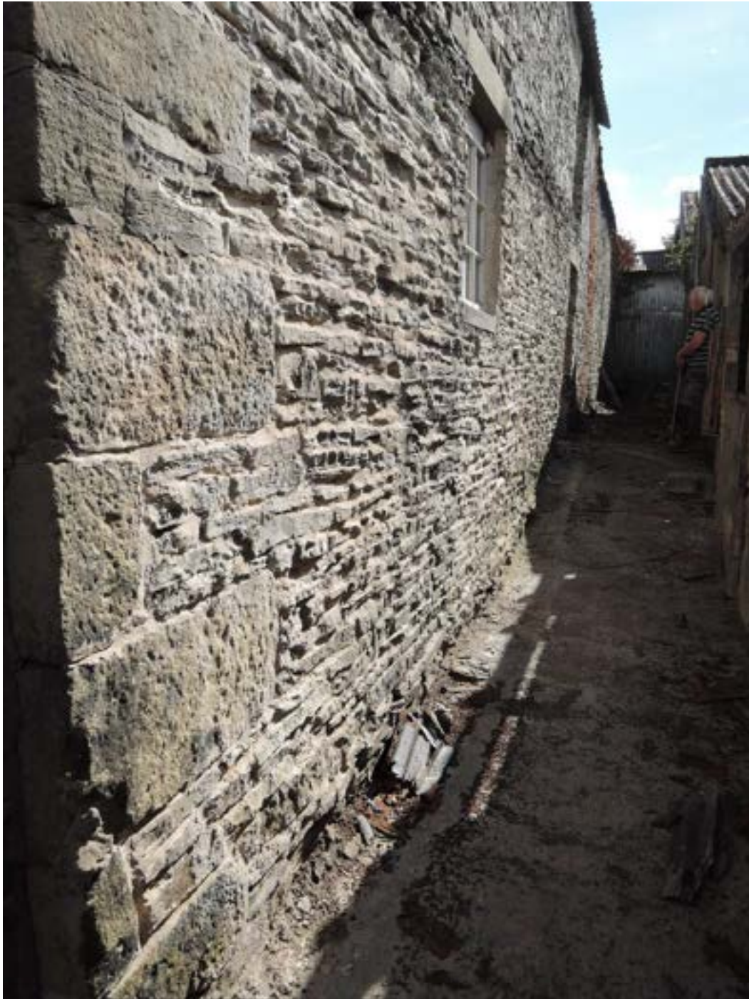
Small barn back wall
