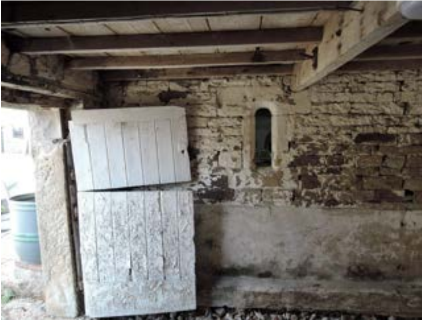
Small barn ground floor party wall with large barn
