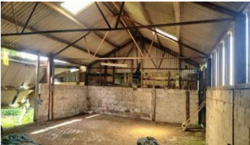
Internal Image of one of the agricultural Buildings to be demolished
