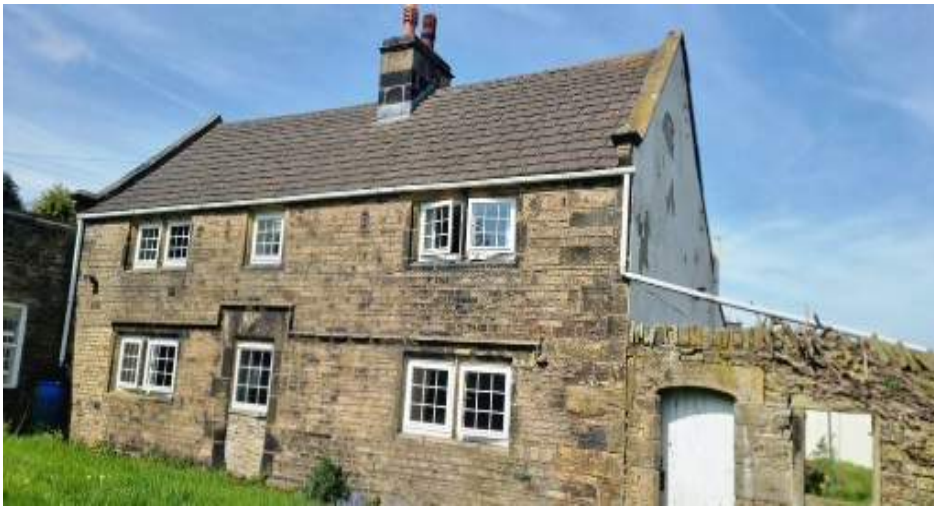
Front Elevation of the Existing Listed Farmhouse
