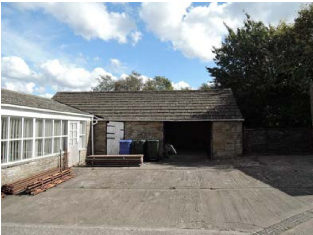
Garage/shed in good order
