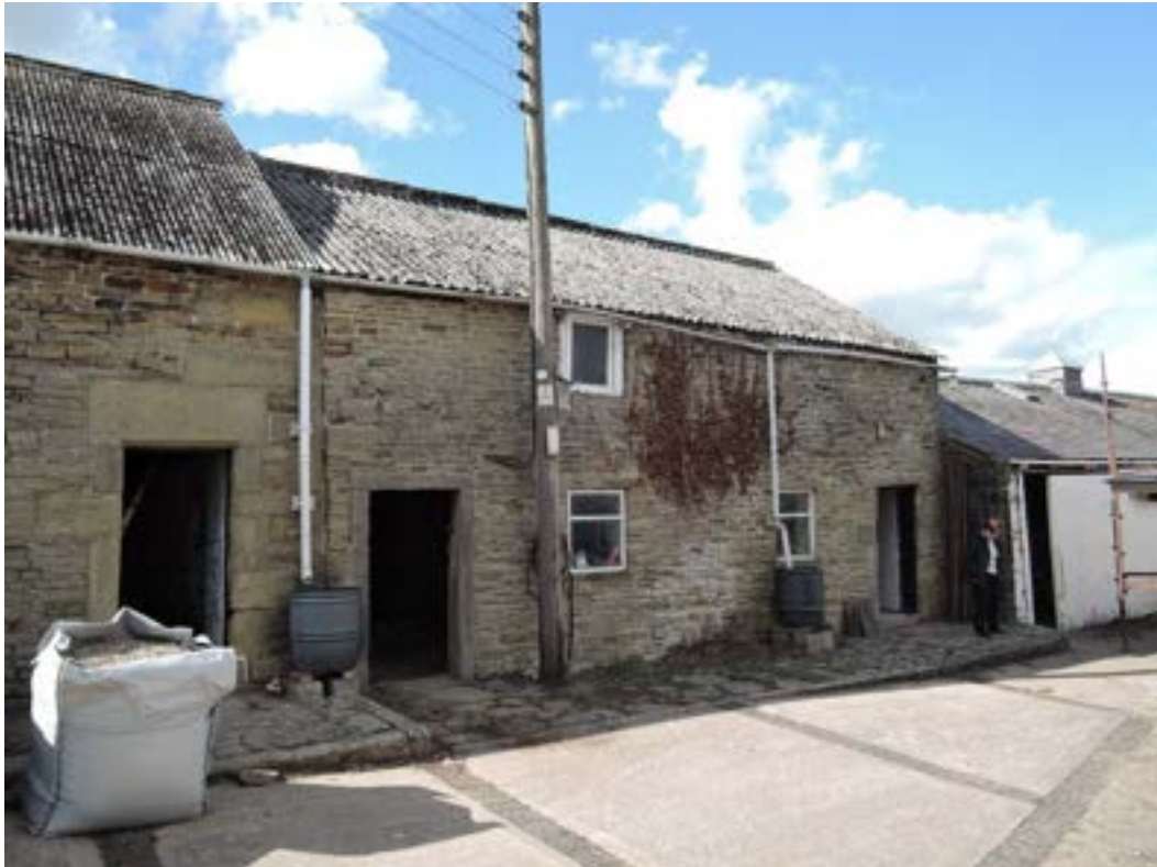
Smaller barn to the north
