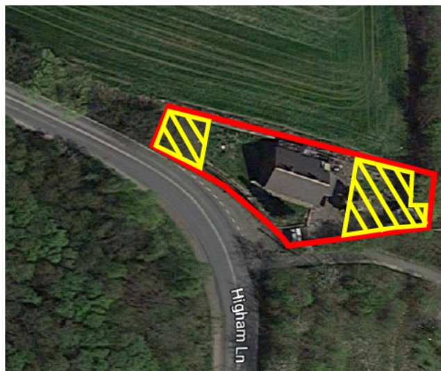
Figure 1: Red line showing bungalow site boundary; yellow hatching showing where demolition/clearance works have taken place to date.
