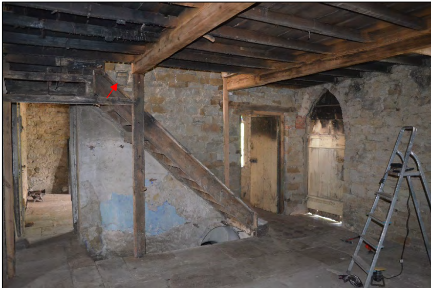
Figure 16: View of ground floor room G1 , looking west indicating location of blocked joist socket.
