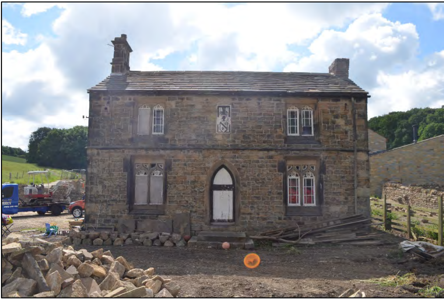
Figure 7: View of the north-east elevation of Bank House
