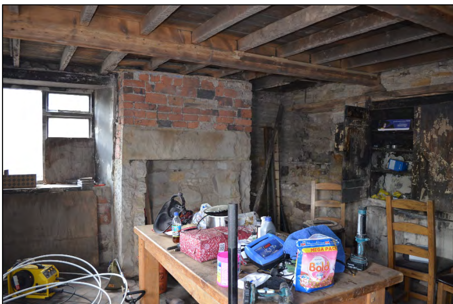
Figure 17: View of ground floor room G3 , looking south
