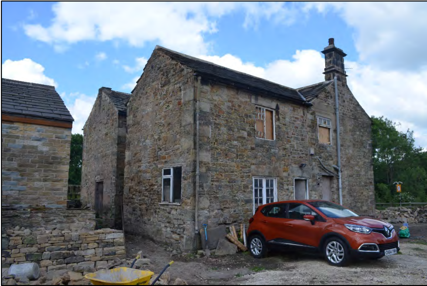
Figure 9: View of the south corner of Bank House
