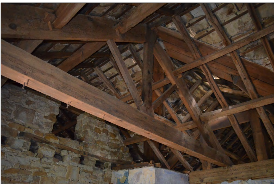
Figure 20: View of the roof structure above first floor room F2 , looking east
