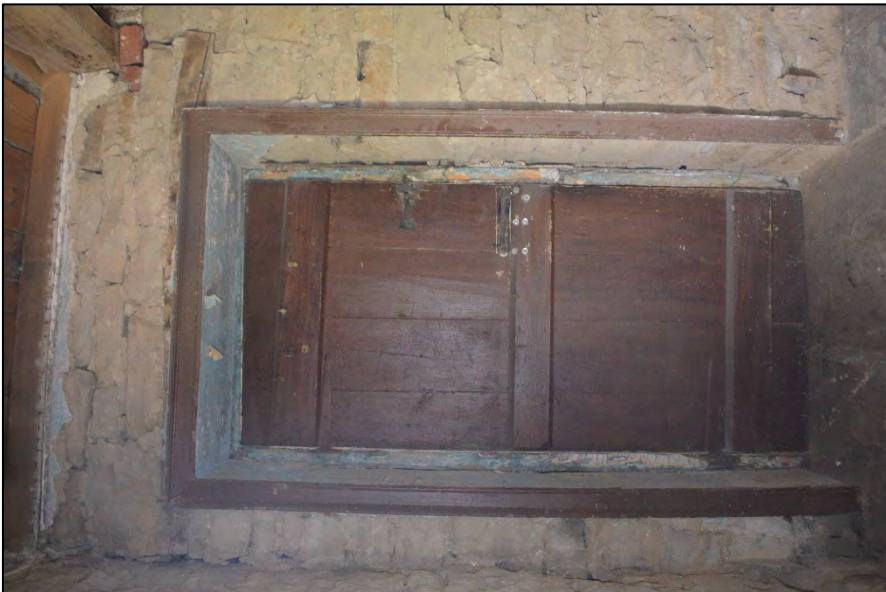
Figure 21: View of plank and ledged door with surround in room G2 , looking north-east
