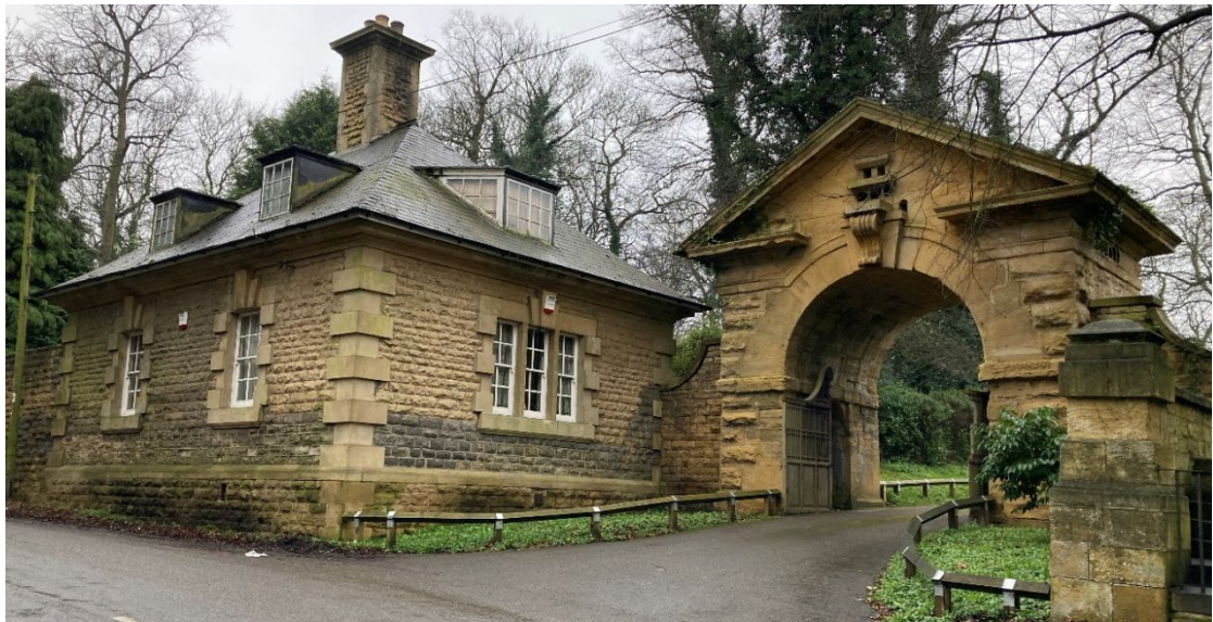
Plate 5 - East Lodge with vertical sliding sash windows
