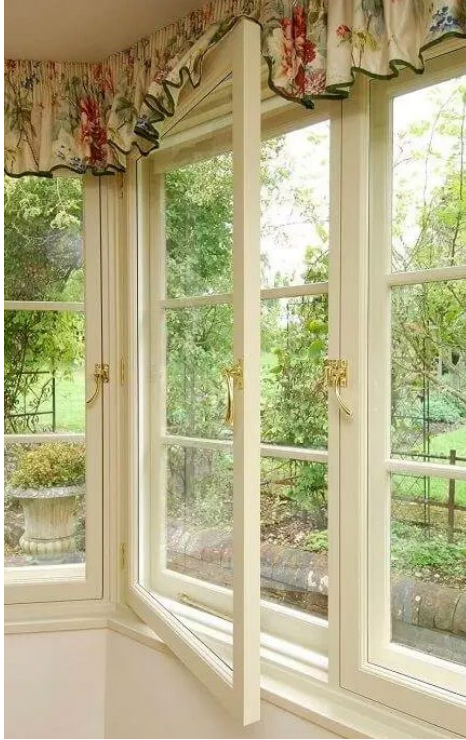
Plate 2 - Timber side hung casement secondary glazing (the Sash Window Workshop)
