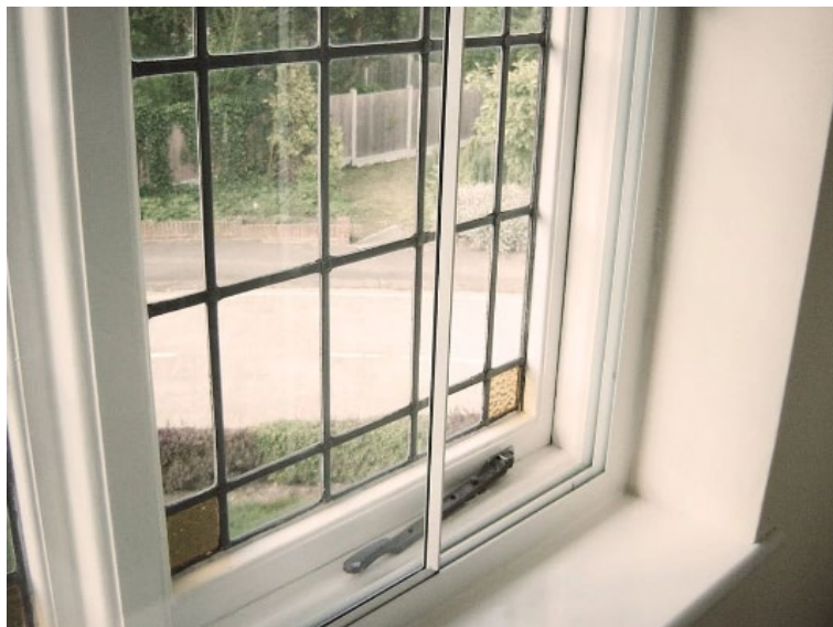
Plate 4 - Aluminium horizontal sash window (elglaze.co.uk)
