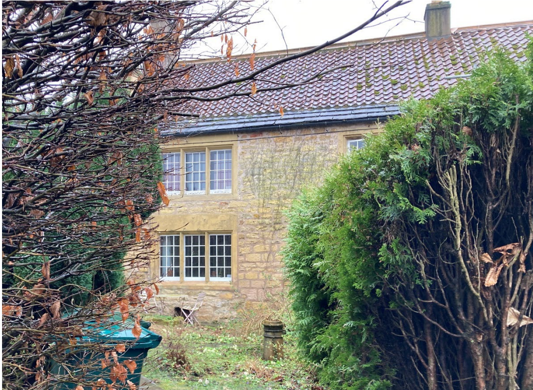
Plate 10 - The windows on the east side of Old School
