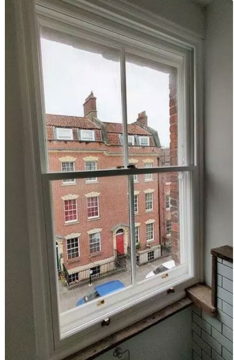
Plate 3 - Timber vertical sash secondary glazing (the Sash Window Workshop)
