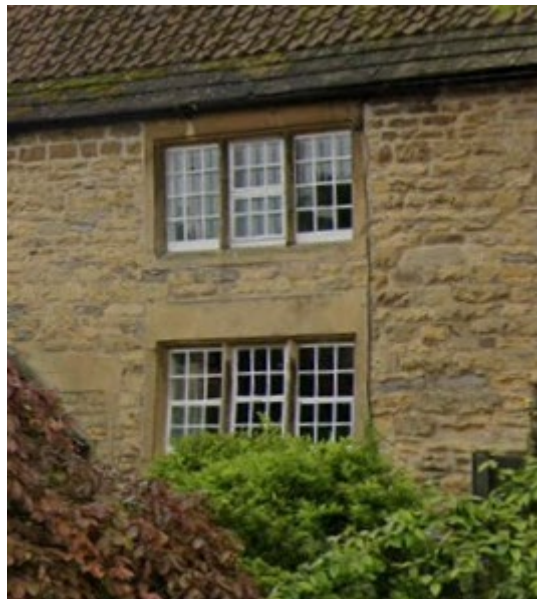
Plate 11 - The windows on the west side of Old School
