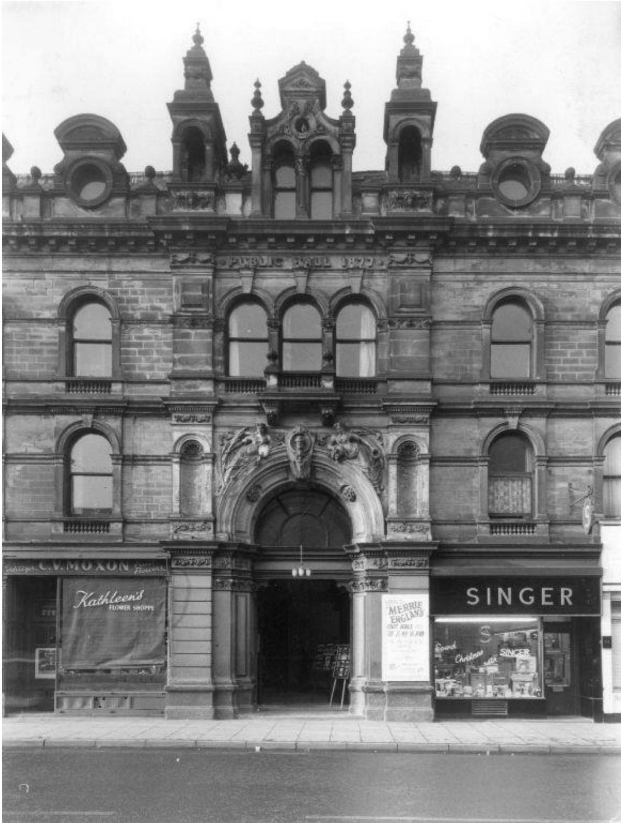
Fig. 24: Archive Image of Entrance 1963
