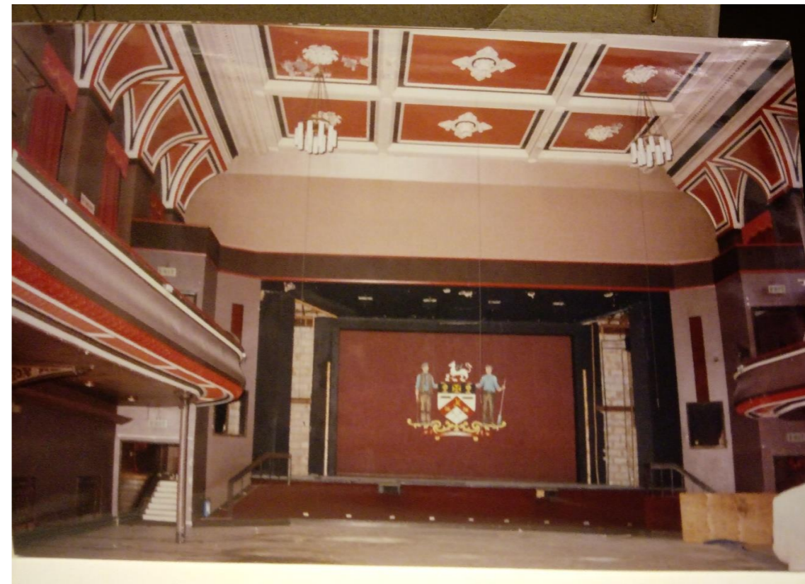
Fig. 26 Below: Archive Photo of the Main Hall circa 1990s
