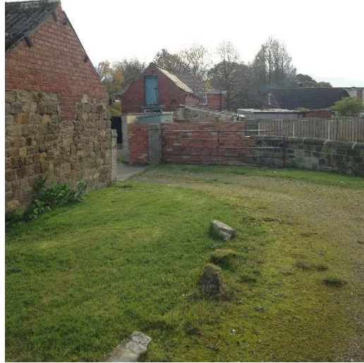
Photograph 1: View looking south towards the main entrance to the site. Note, to the rear of the photograph, a small double storey outbuilding. Unable to access this building as it was not structurally safe.
