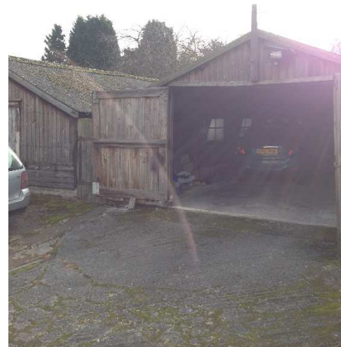
Photograph 5: View looking south into the single storey outbuildings now used as garages. The floor slab was noted as being in good condition with no obvious signs of fuel or oil spillage.
