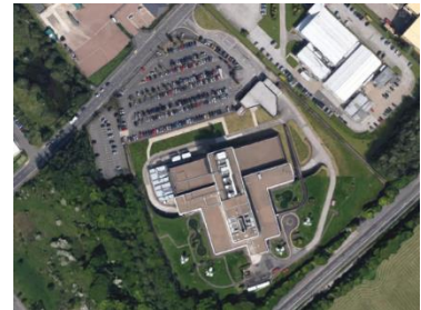
Figure 1 | SYGDC Tankersley, South Yorkshire (image from Google maps)
