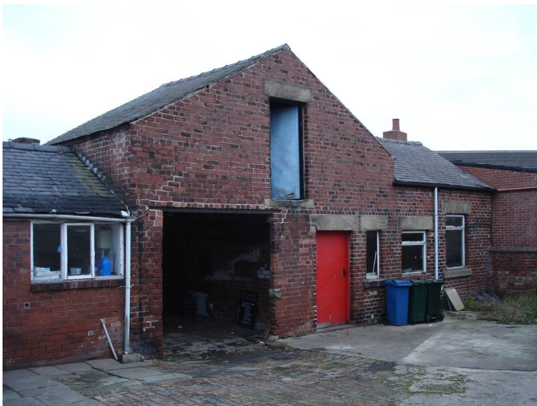
Views of outbuildings to rear.
