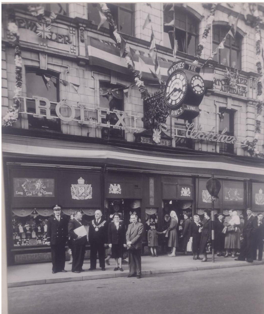
Fig 03. Historic photograph of the Harral Building covered with bunting and flags for the Chamber of Trade Shop Decoration Competition on the 29 th May 1953 (reproduced with kind permission of the Barnsley Archives).
