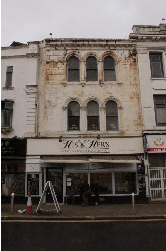
Fig 05. The central stone block on the Eldon Street frontage
