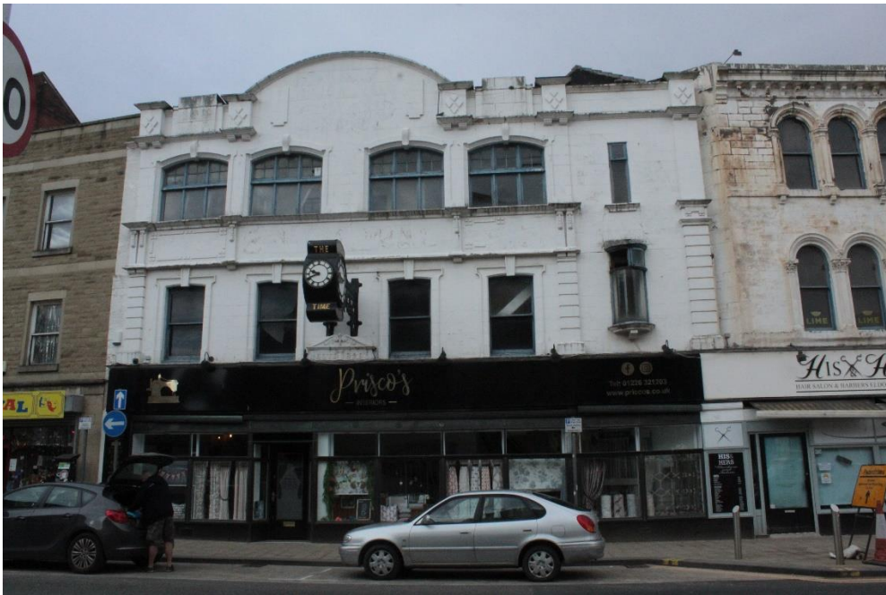
Fig 21. The Eldon Street frontage of no. 32 at the western end of the Harral Buildings.
