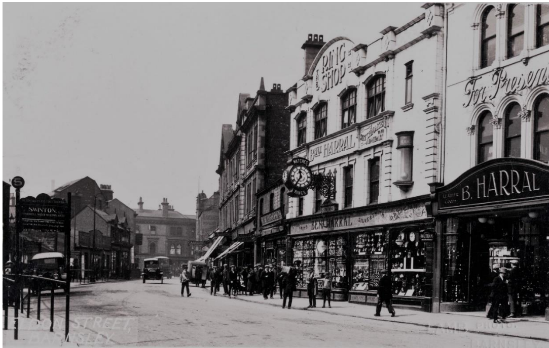
Fig 04. Historic photograph of the Harral Building from the 1920s showing the faience lettering to the arched pediment (reproduced with kind permission of Barnsley Archives).
