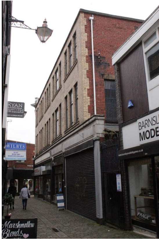
Fig 08. The Arcade elevation of the easternmost block (looking towards Eldon Street)
