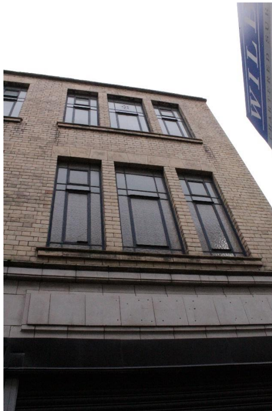
Fig 09. The windows along the Arcade elevation are triple grouped in a Venetian style
