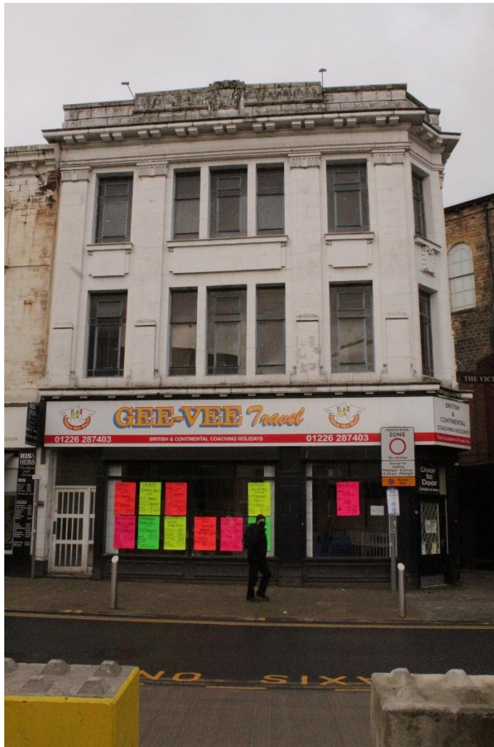
Fig 25. The Eldon Street frontage of no. 36-38 at the eastern end of the Herral Building.
