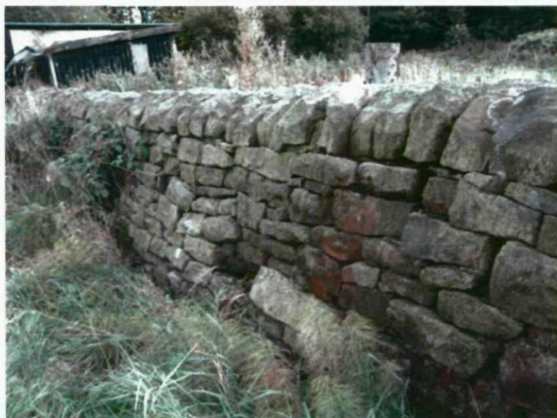
A dry stone wall surrounds the site. This is suitable for common lizards if present.
