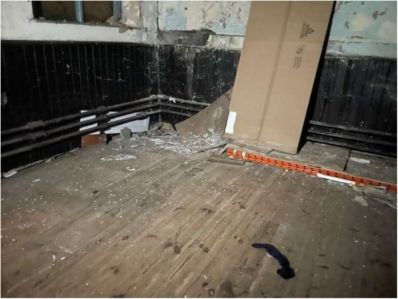
Upper floor front room
