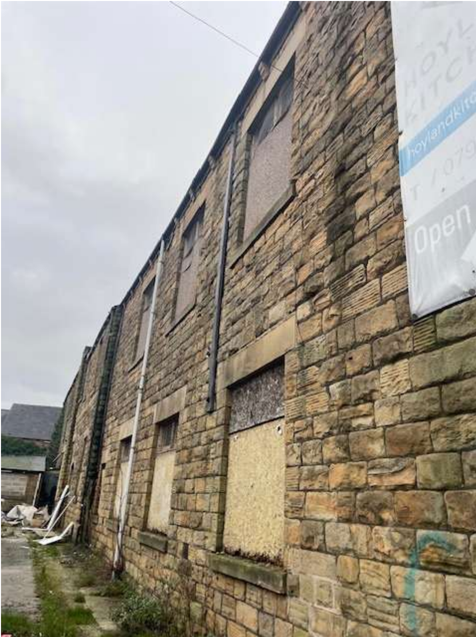
Ties to provide structural stability
