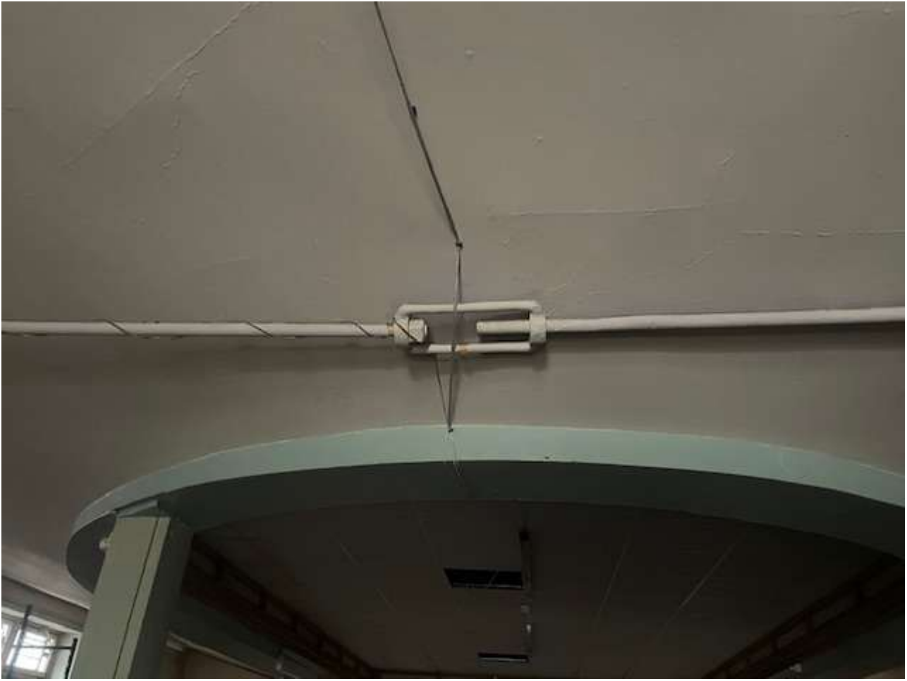
Ground floor front room
