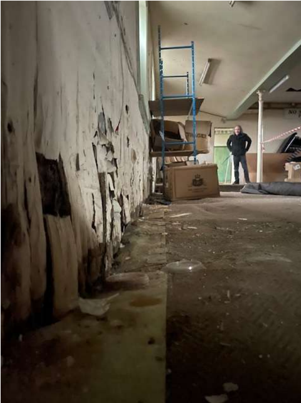
Ground floor room
