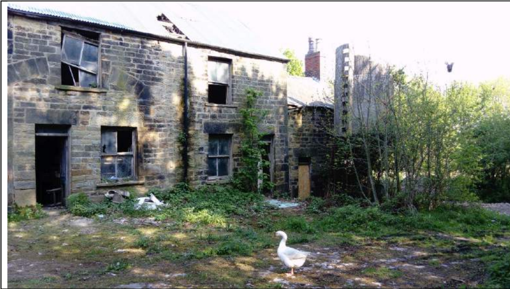
Derelict cottages in northern portion of the site
