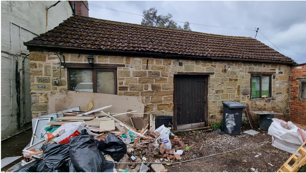
Outbuilding to be demolished as per previously approved application 2018/0716
