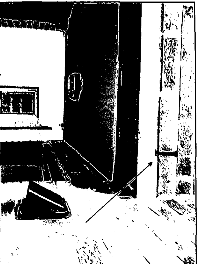
Missing mortar
