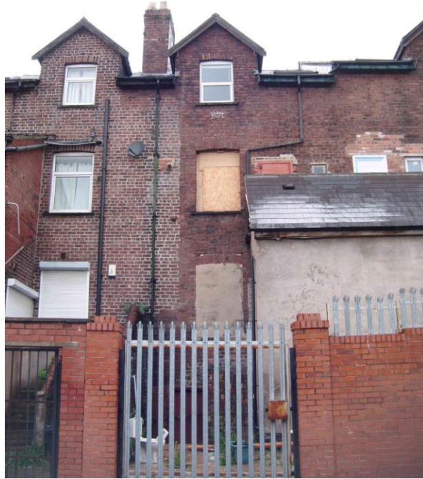
Figure 4 – View of rear elevation no. 49
