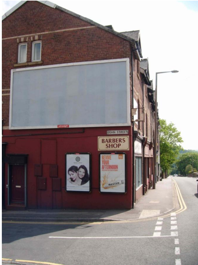
Figure 7 – View looking south along Park Road
