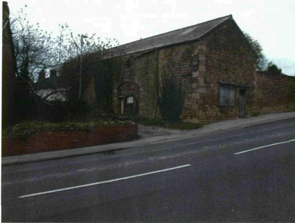
5. The two storey stone barn viewed from the South West.
