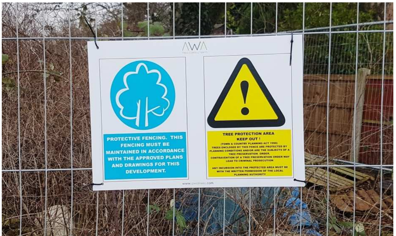
Figure 5: Example of A3 Correx Tree Protection Warning Sign fixed to fencing panel
