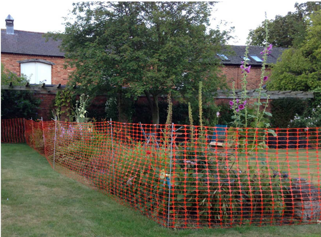
Figure 3: Plastic mesh fencing secured with heavy duty metal stakes
