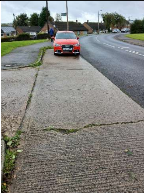
Lay-by deterioration.
