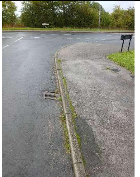
Photo 9 Saville Road / Gilroyd Lane
