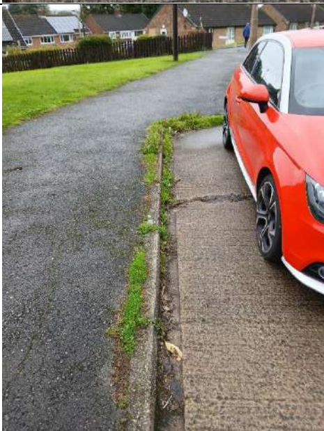
Lay-by deterioration.
