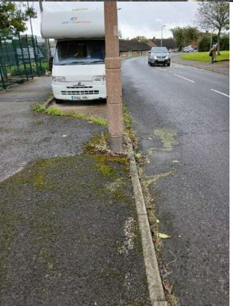
Footway deterioration.
