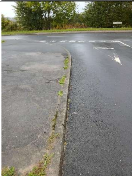
Photo 8 Saville Road / Gilroyd Lane
