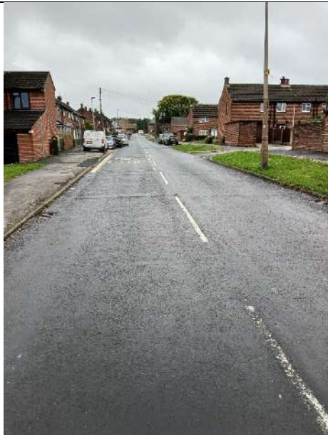
Photo 7 Saville Road / Gilroyd Lane
