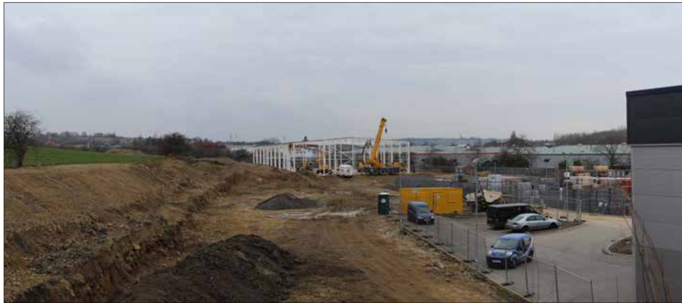
Onsite Viewpoint 1: Looking in a westerly direction across the site.
