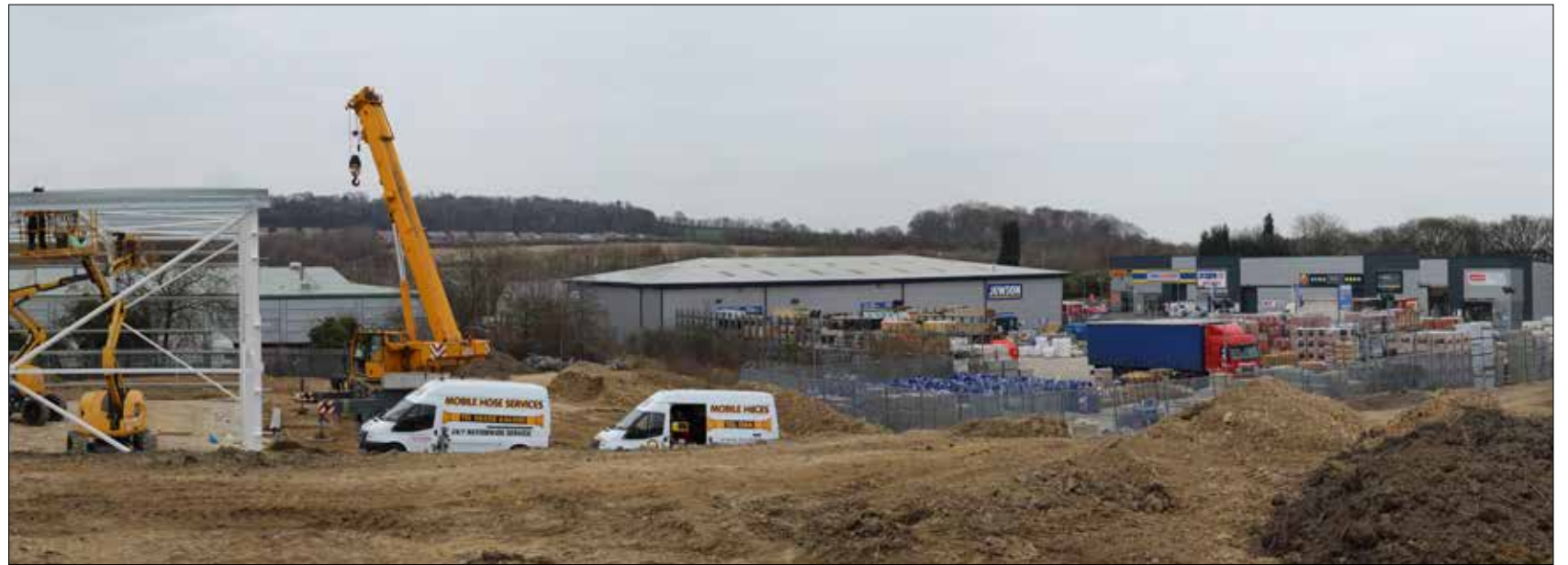
Onsite Viewpoint 5: Looking in a northerly direction.
