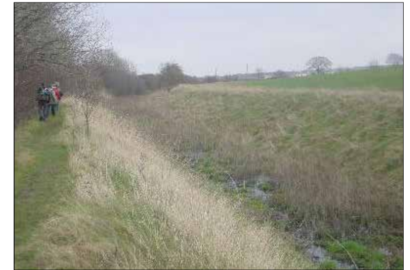
There is a small amount of water in the canal bed.
