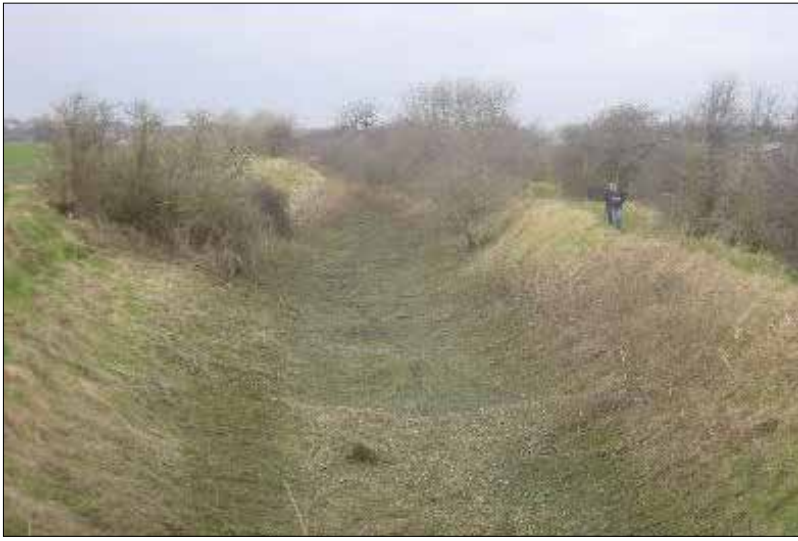
Looking West from Caulk Lane towards Stairfoot. The canal channel is intact but dry.
