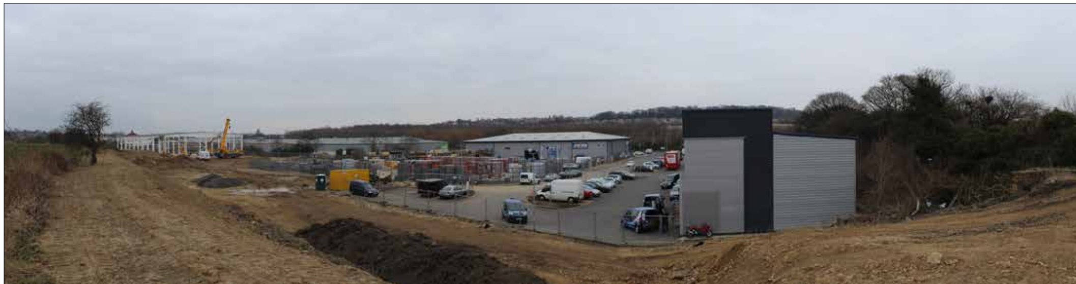
Onsite Viewpoint 2: View from top of embankment looking west.
