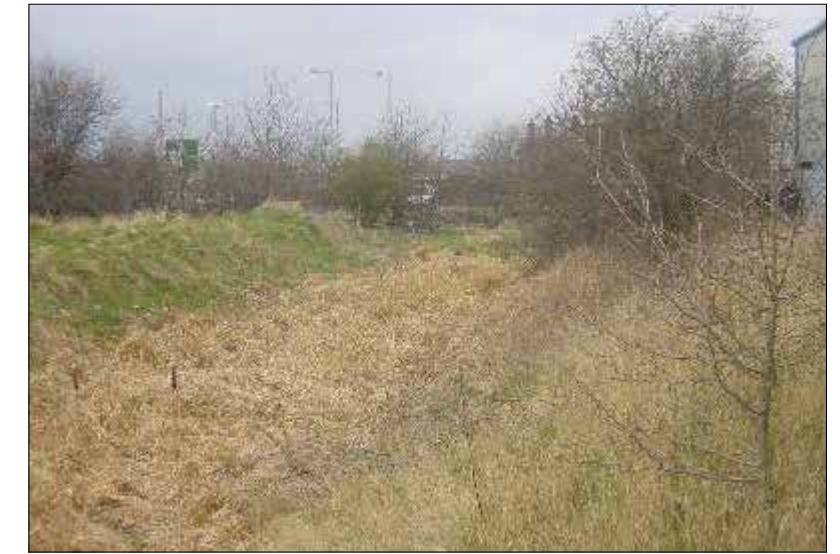
Approaching the one way traffic system at Stairfoot. Beyond Bleachcroft Way, the canal has disappeared under the new alignment of Doncaster Road
