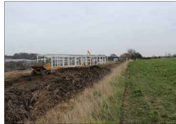
Onsite Viewpoint 7: View from west of site looking east.
