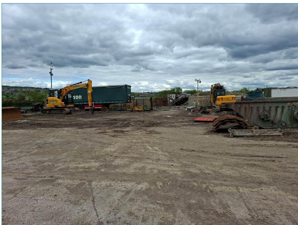
Photograph 10: Wordsworth Compound Looking Northeast, Crushing Area.
