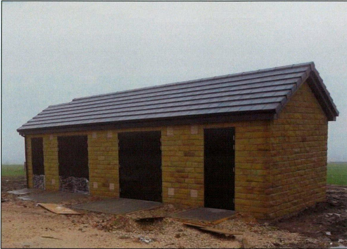
Figure 2.8 – Existing Spicer Hill sub-station.
