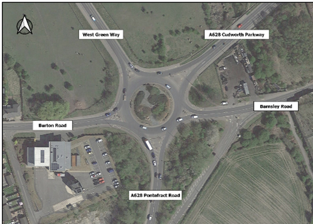
Figure 3-8 A628 Pontefract Road / West Green Way / Burton Road Roundabout
