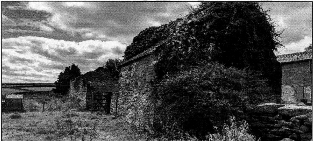
Plate 3. Example of open joints and access to wall top on B1
