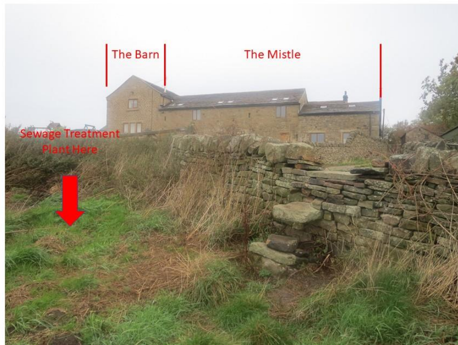
View to The Mistle (looking North West)
