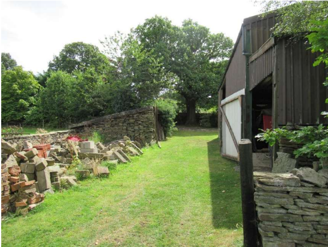
Photograph 1 – Looking south between the lean-to and barn.
