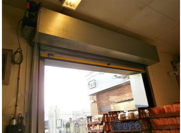
Roller shutter No. 10 – Internal (External View)
