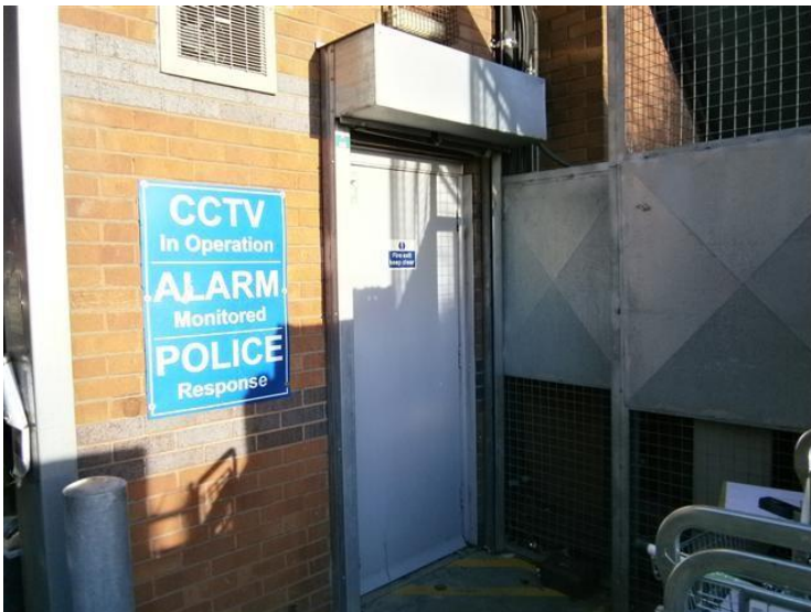
Roller shutter No. 11 - External
