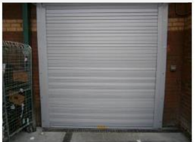
Example of External shutter after – Use of solid slats
