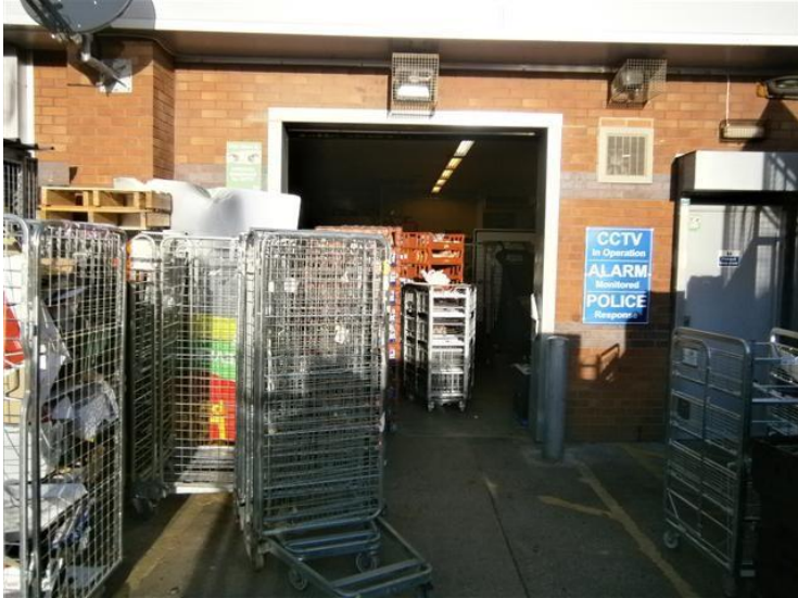
Roller shutter No. 10 – Internal (External View)
