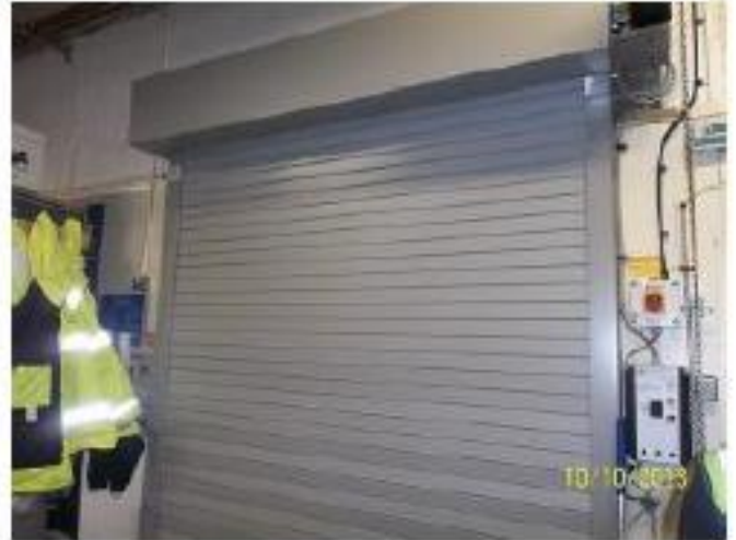
Example of internal shutter after – Use of solid slats
