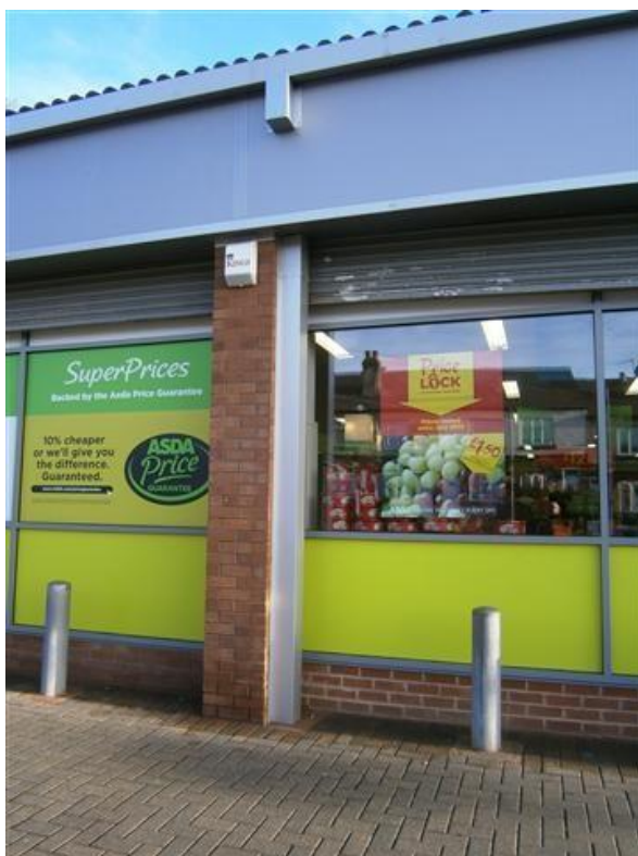
Roller shutter No. 7 & 8 - Concealed
