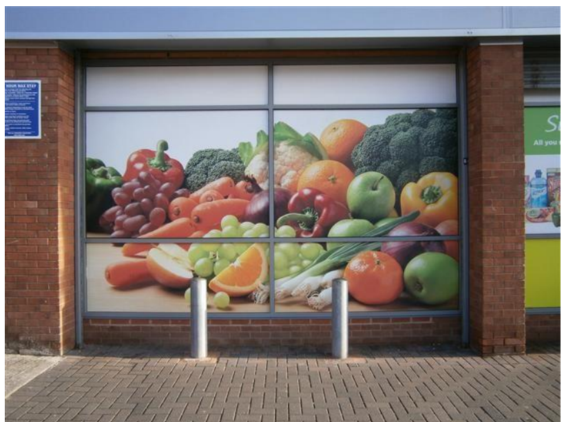
Roller shutter No. 9 - Concealed
