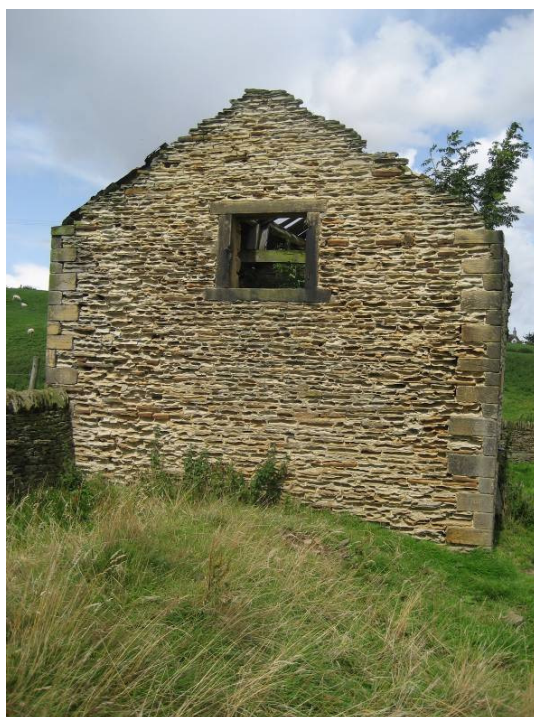
5. South west gable
