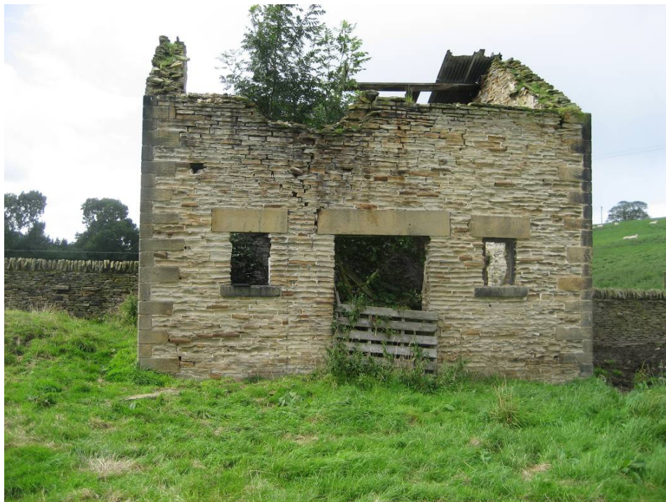
4. South east elevation of redundant field barn set within the north west corner of the field against existing field boundary walls.
