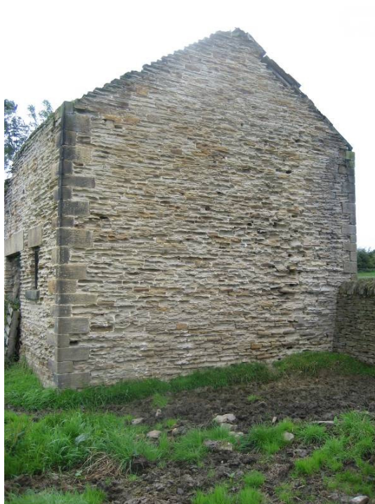
6. North east gable
