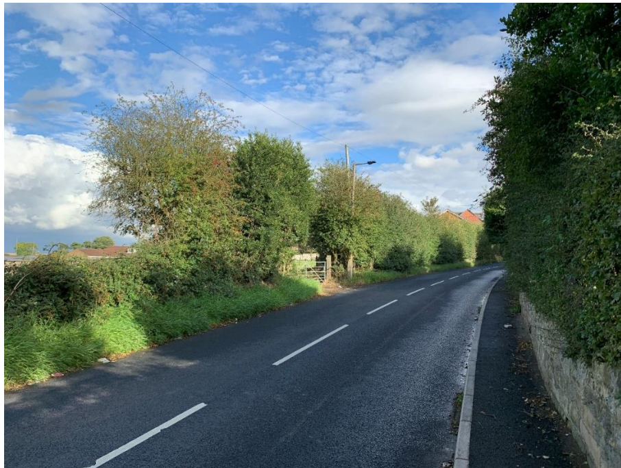
Photograph 2: Site access point in direction of Barnsley Road
