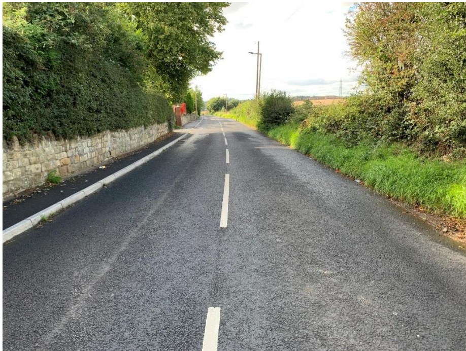
Photograph 3: Site access in the direction of South Hiendley
