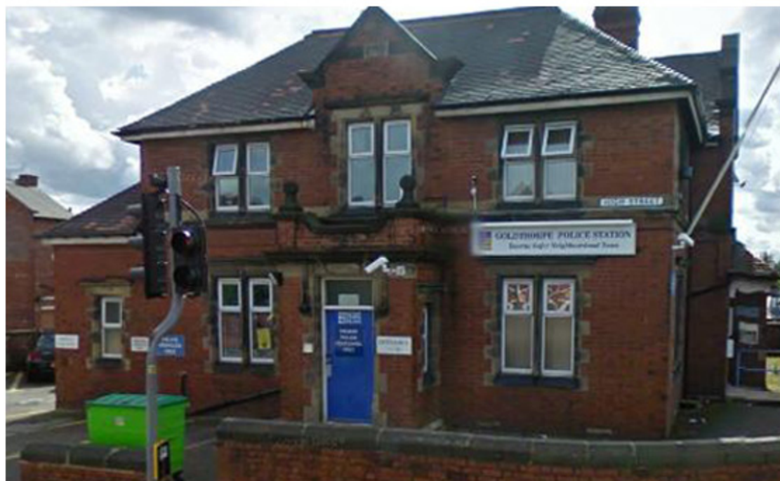
Goldthorpe Police Station: As existing
