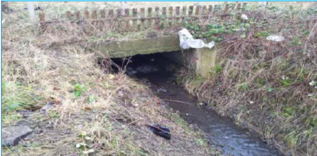
Figure 1 - Downstream Face 1 (on site)
