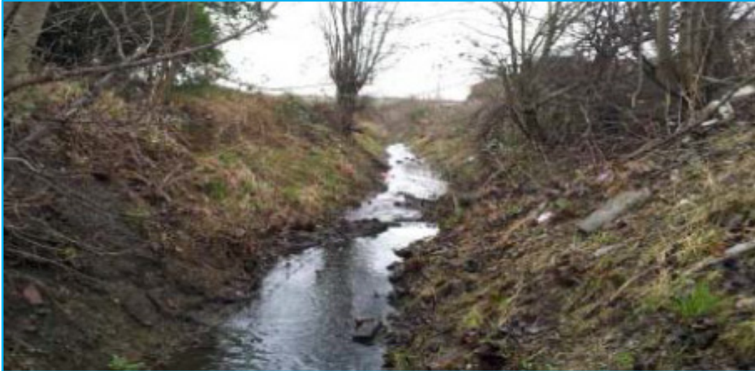
Figure 4 - Channel Downstream of Culvert
