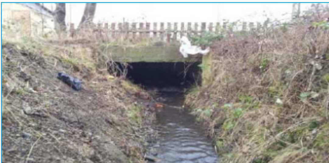
Figure 2 - Downstream Face 2 (on site)
