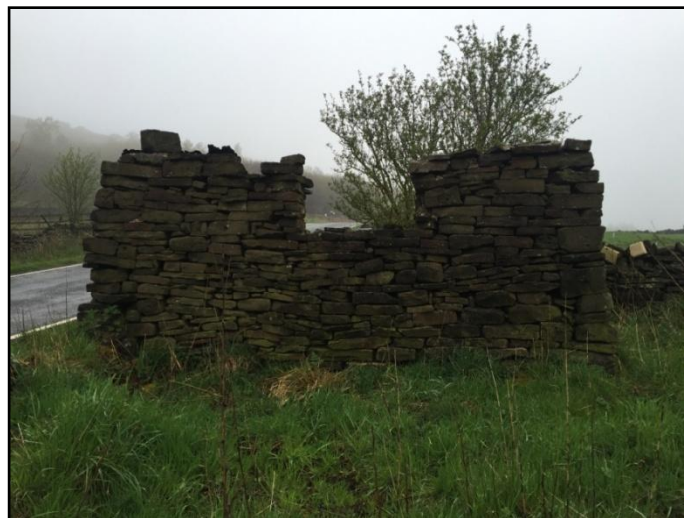
Figure 10. Second building on site.
