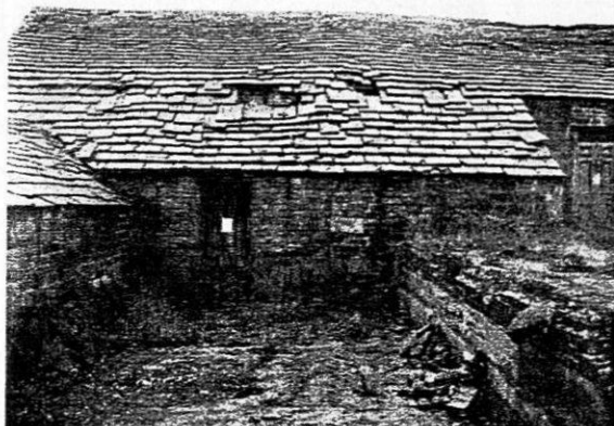
Fig 18 Cat slide roof to the rear of Barn B
