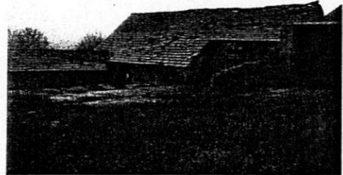
Fig 12 North and east elevation – Barn B
