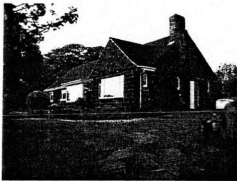
Fig 1 South and east elevation of bungalow
