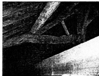
Fig 14 Half truss from timber post
