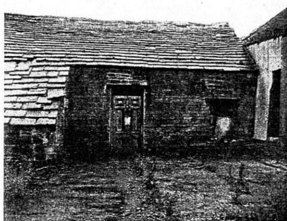
Fig 17 East elevation – Barn B – north end
