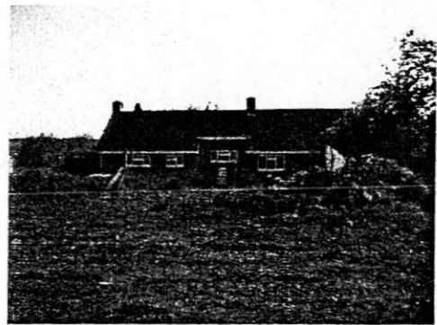
Fig 2 North elevation of bungalow
