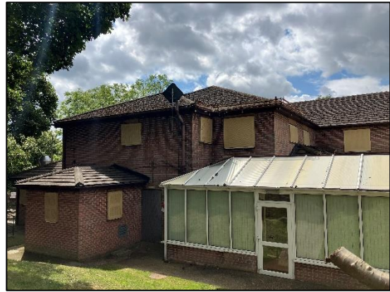
Figure 24: B2's northern aspect, view looking south.
