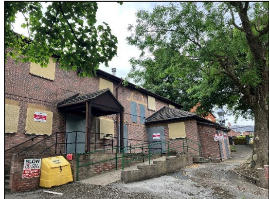
Figure 28: View of B2 porch and eastern-facing single-storey extension.
