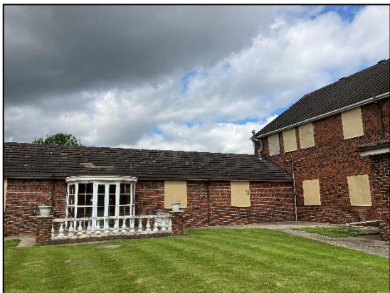
Figure 21: Internal courtyard – western view of B1.
