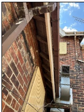
Figure 19: View of PRF-I on B1 northern single-storey extension.
