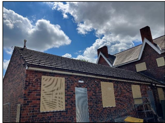
Figure 16: B1 single-storey northern extension, (view from the north, looking south).
