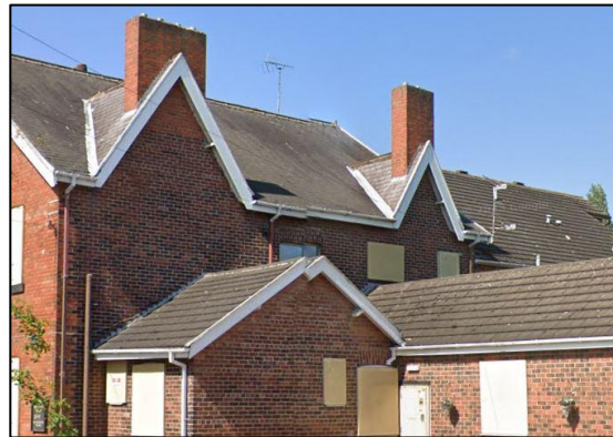
Figure 18: The northern gable ends, viewed from the northern entrance/vehicle access (looking southwest).
