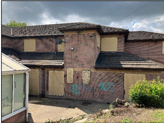
Figure 25: View of B2, another northern aspect, view towards the south.
