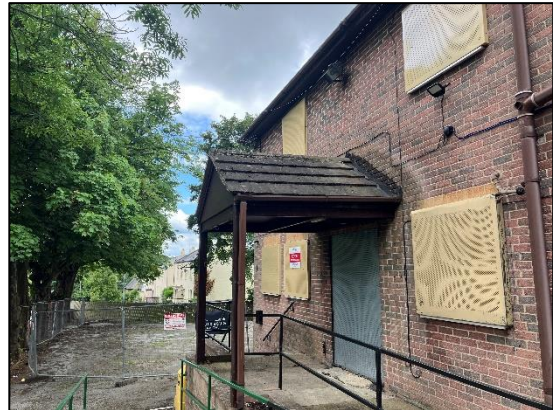
Figure 26: The rooftop porch of B2, eastern aspect.
