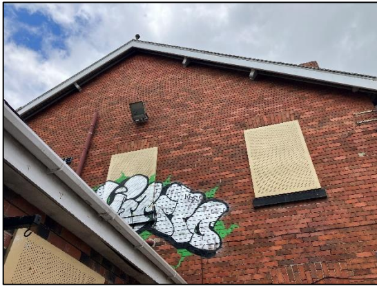
Figure 23: B1 northeastern gable-end; sealed and intact.
