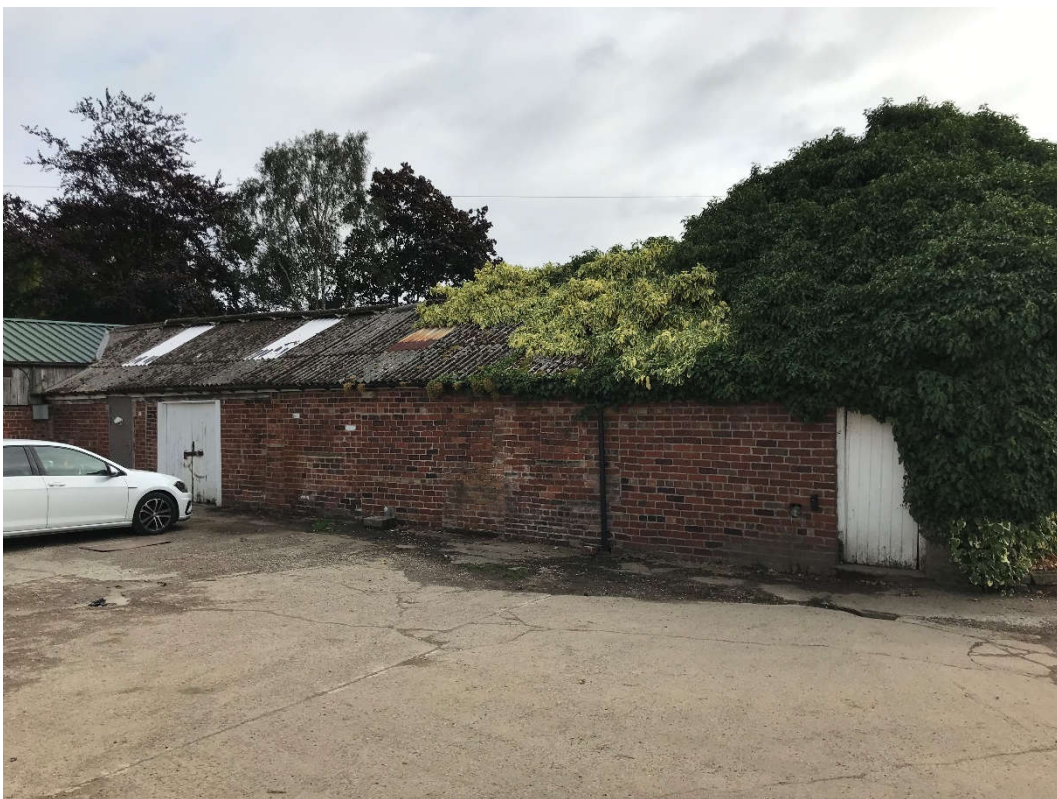
Fig 02. Existing outbuilding west elevation.
