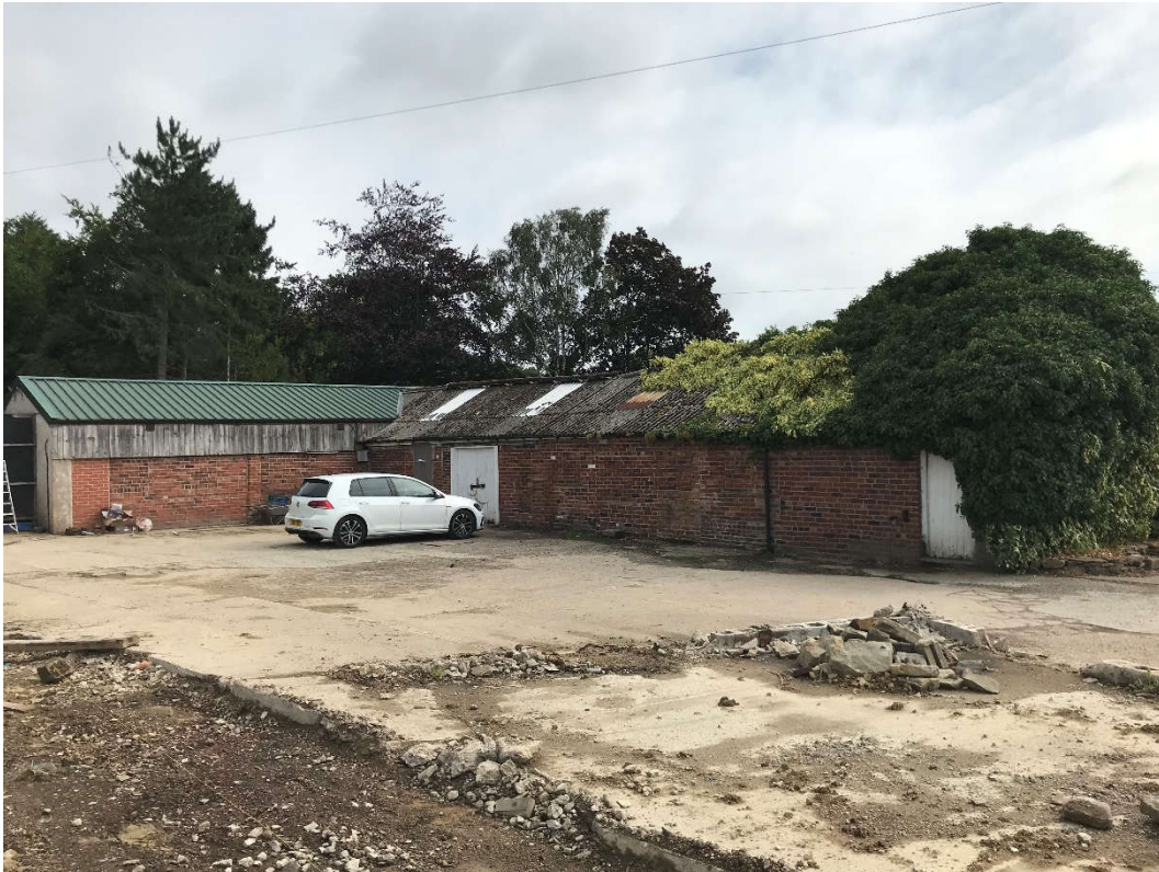
Fig 01. View of south and west elevations of outbuildings looking north east.
