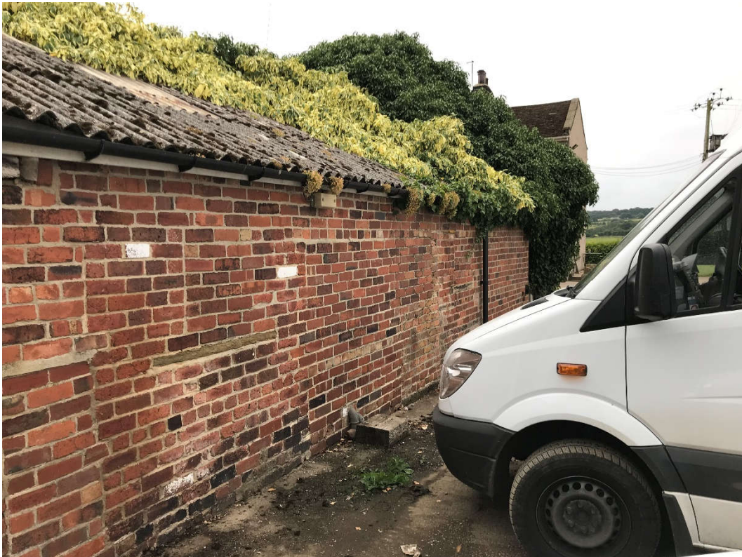
Fig 05. East elevation of outbuilding showing original pier and openings altered.
