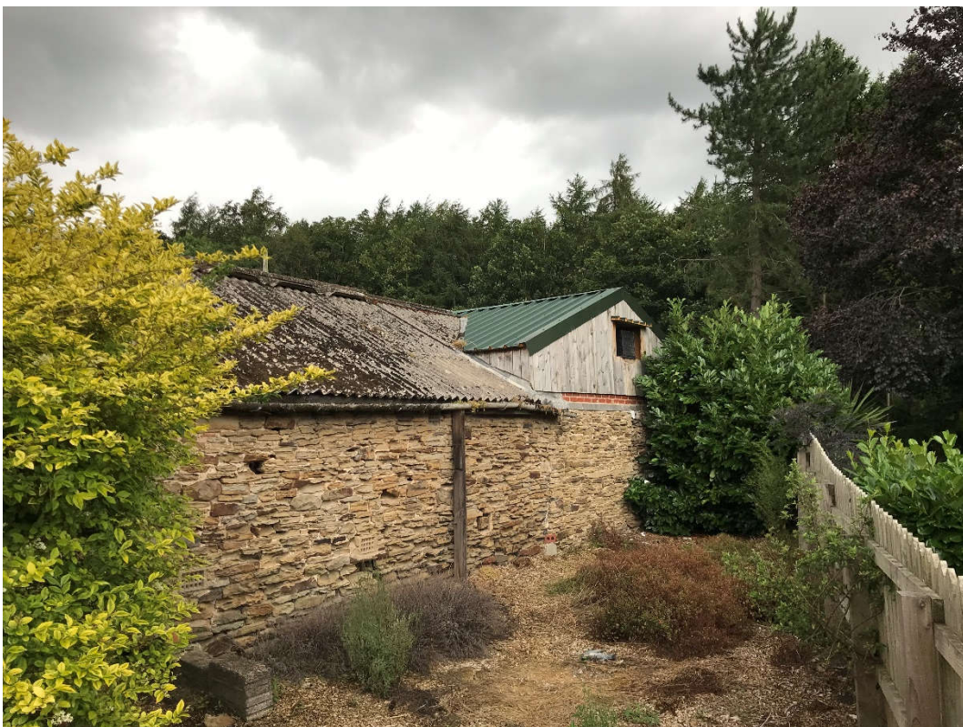
Fig 06. Rear of outbuilding. East elevation in natural stone.
