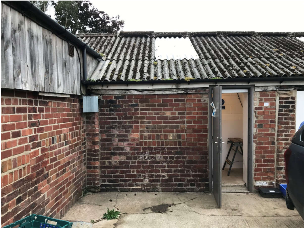
Fig 03. Extg outbuilding showing original brick piers and eaves beam.
