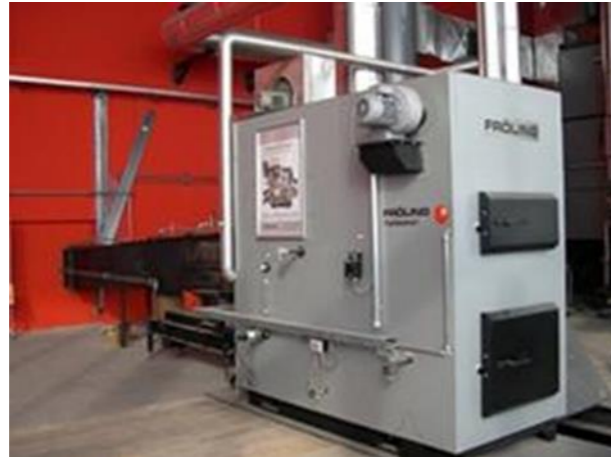
Figure 13 – Biomass Boiler
