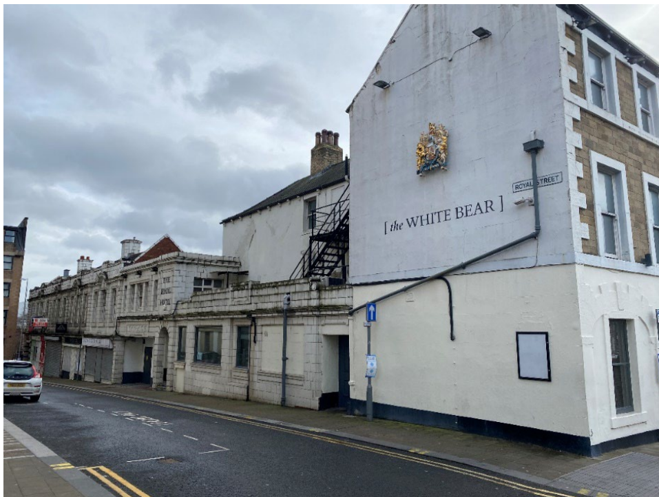
1.1 View from Church Street down Royal Street before completion
