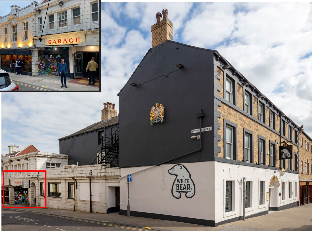
1.4 Photograph showing the existing pub after completion, with red box showing where the street art locates
