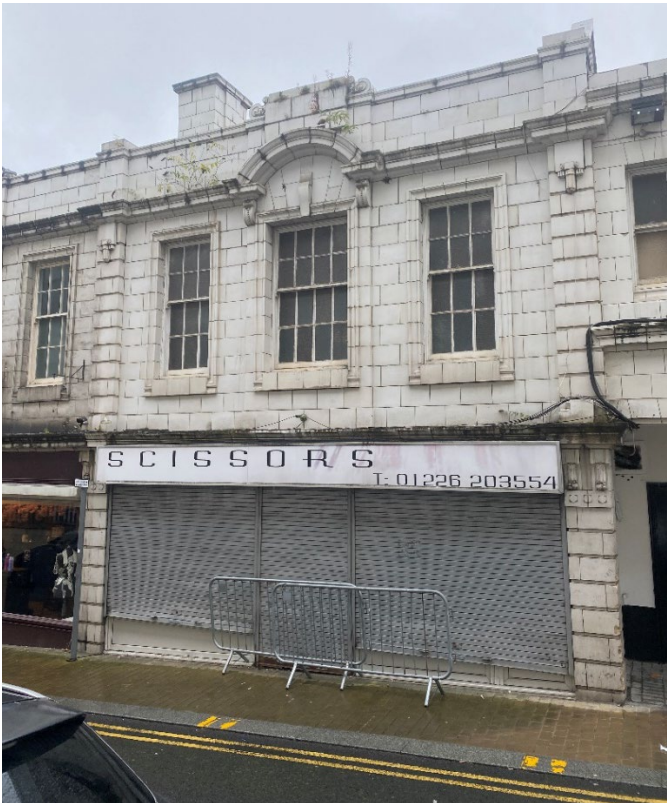
1.3 Current redundant shop unit with security shutters and Function Room over
