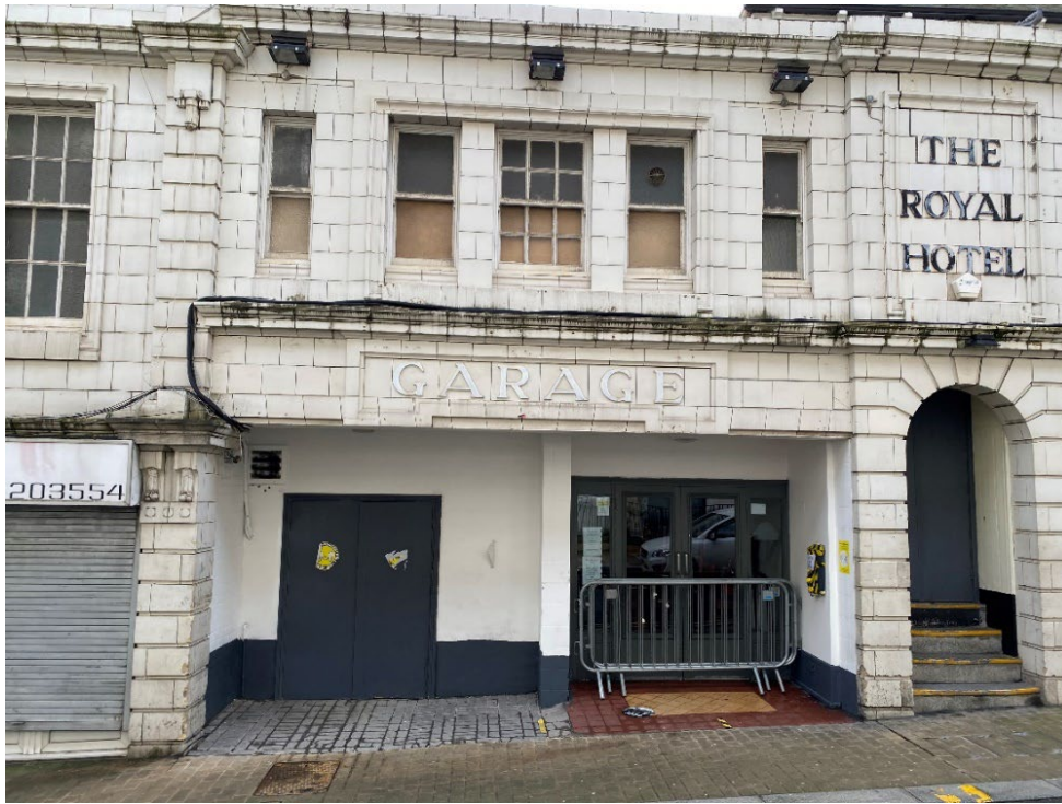
1.2 View from Royal Street – existing rear entrance before completion
