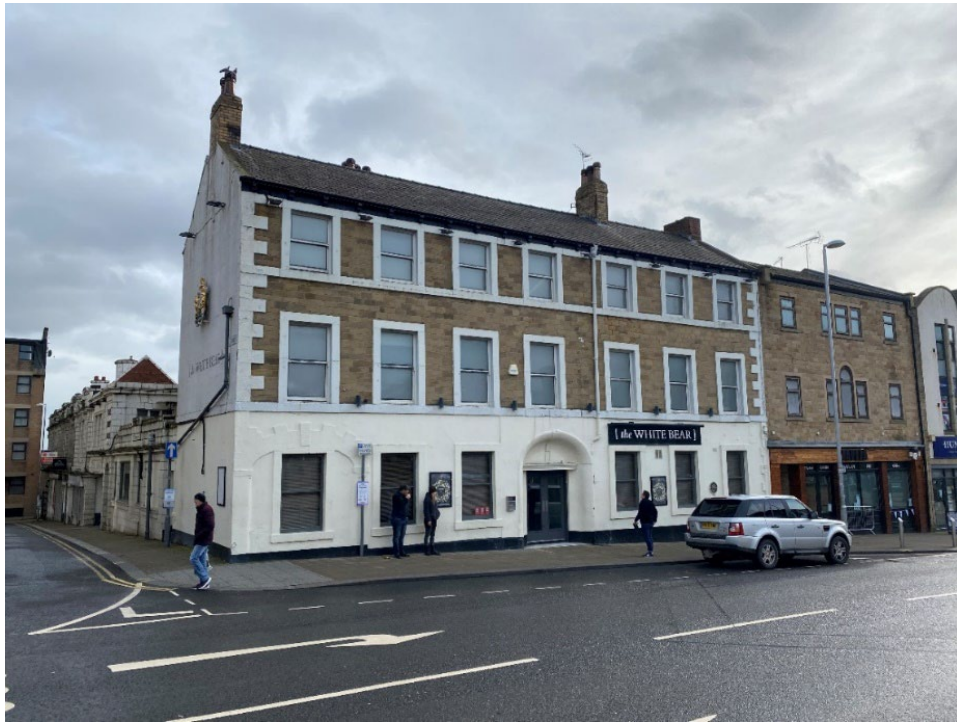
1.0 Front façade from Church Street before completion
