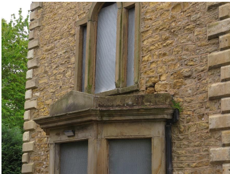
Fig 7 – Bay Window with venetian window over
