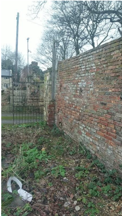
Fig 10 – NorthE boundary – brick
