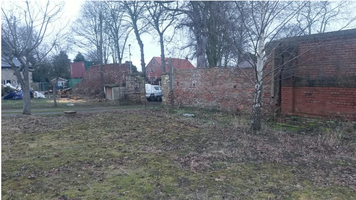
Fig 8 –North boundary – clay brick; stone gateposts; engineering brickwork
