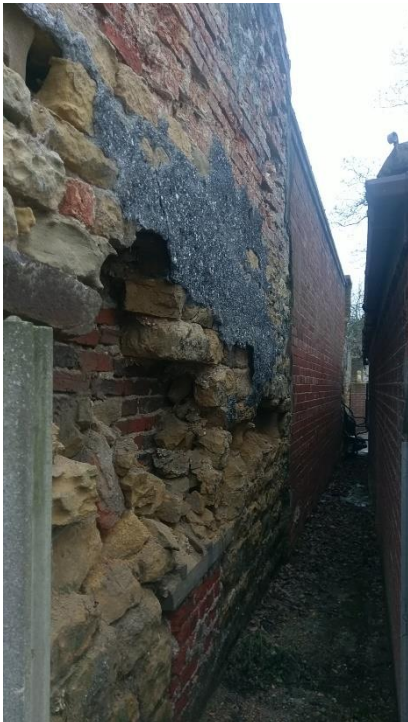
Fig 12 – NE boundary – brick and stone.
