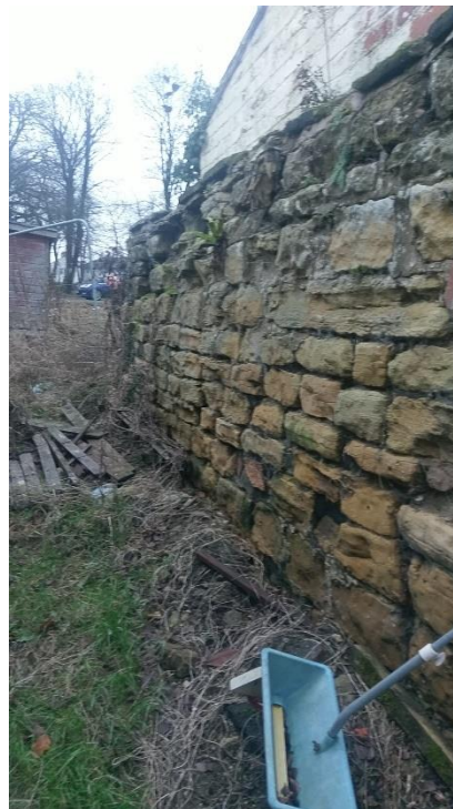
Fig 13 – NE return – stone outer facing
