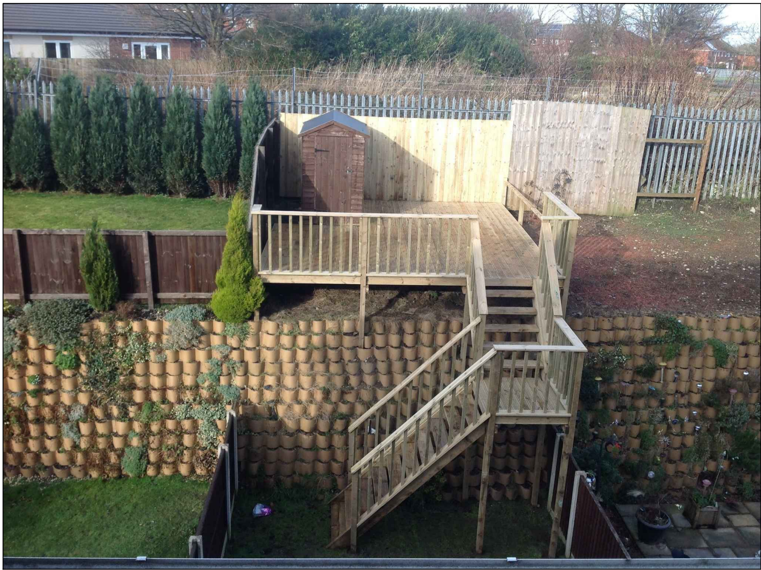
As Existing South Facing Elevation Photograph Taken 1st February 2014
