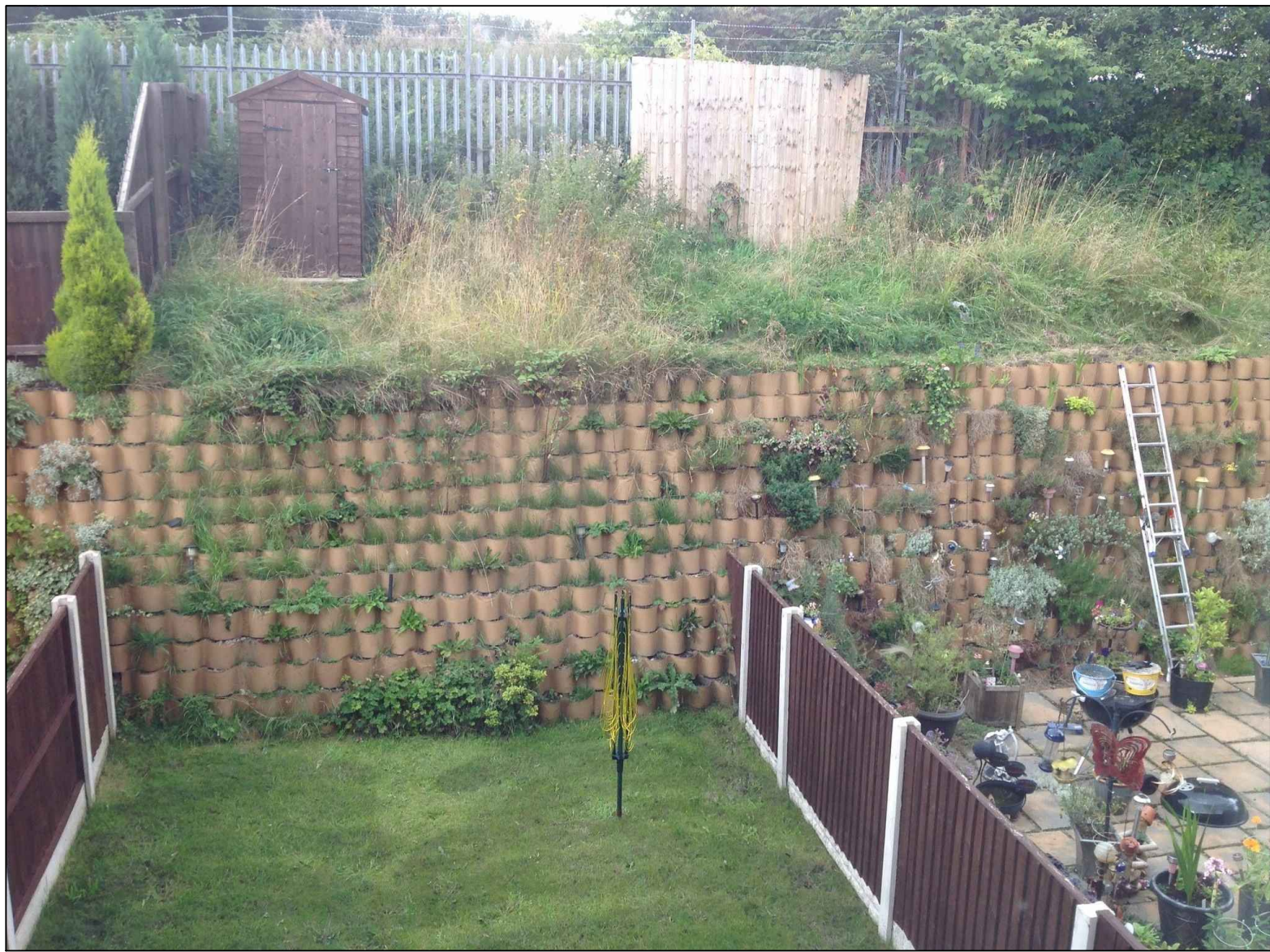
Original South Facing Elevation Photograph Taken 14th September 2013
