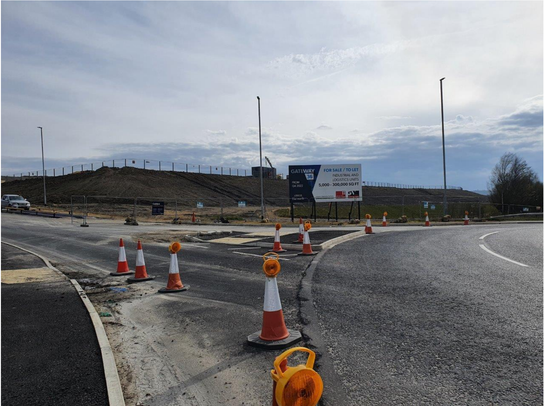
Photograph 1. 'Sign 1' (already installed). Date: 11 April 2022.
