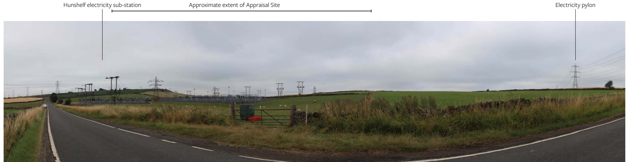
Viewpoint 1 - View looking south east towards the Appraisal Site from Tofts Lane. There are open views to the Appraisal Site, including portions of the pastoral field ground plane and the boundary dry stone wall. The site is viewed in the context of the nearby energy infrastructure elements including a number of nearby electricity pylons and the vertical elements of Hunshelf electricity sub-station.
