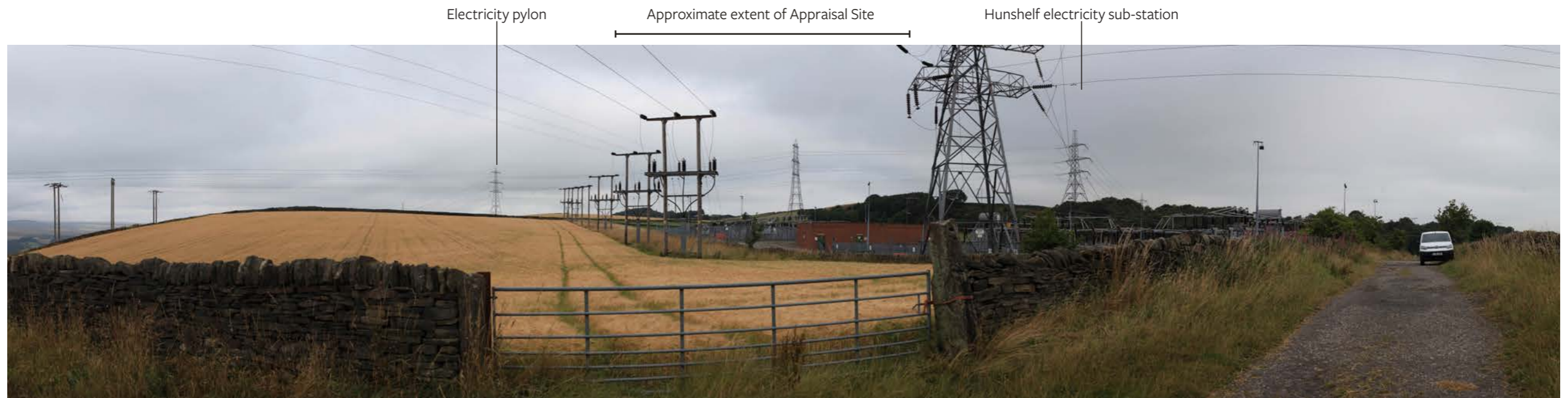
Viewpoint 4 - View looking north west towards the Appraisal Site from Footpath BL|Hunshelf CP|33, Mucky Lane. There are partial glimpsed views to the Appraisal Site, through and above the vertical elements of Hunshelf electricity sub-station.
