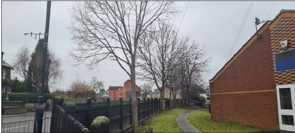
External inspection – care home
