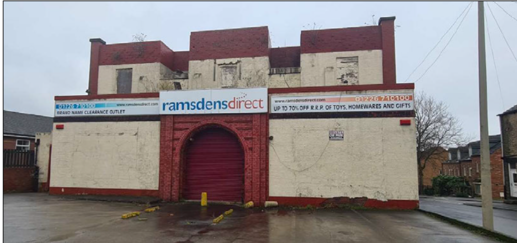
Plate 5. The façade of the former cinema (viewed from the west)
