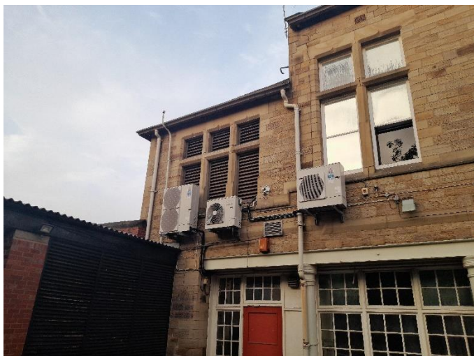
Figure 7 Louvre vents on western and northern elevations.
