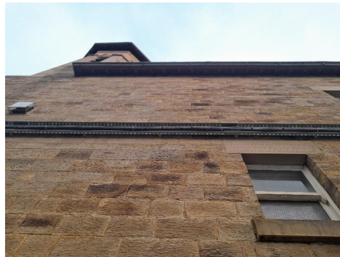
Figure 8 Duct and vented window on northern elevation.
