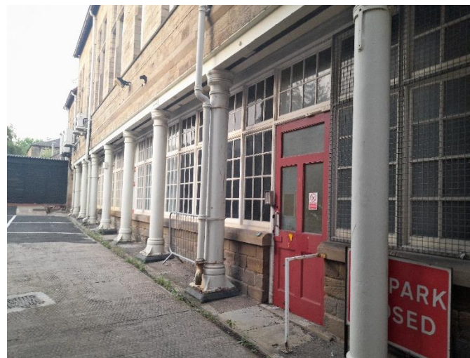
Figure 6 Colonnade; gaps between metal beams.
