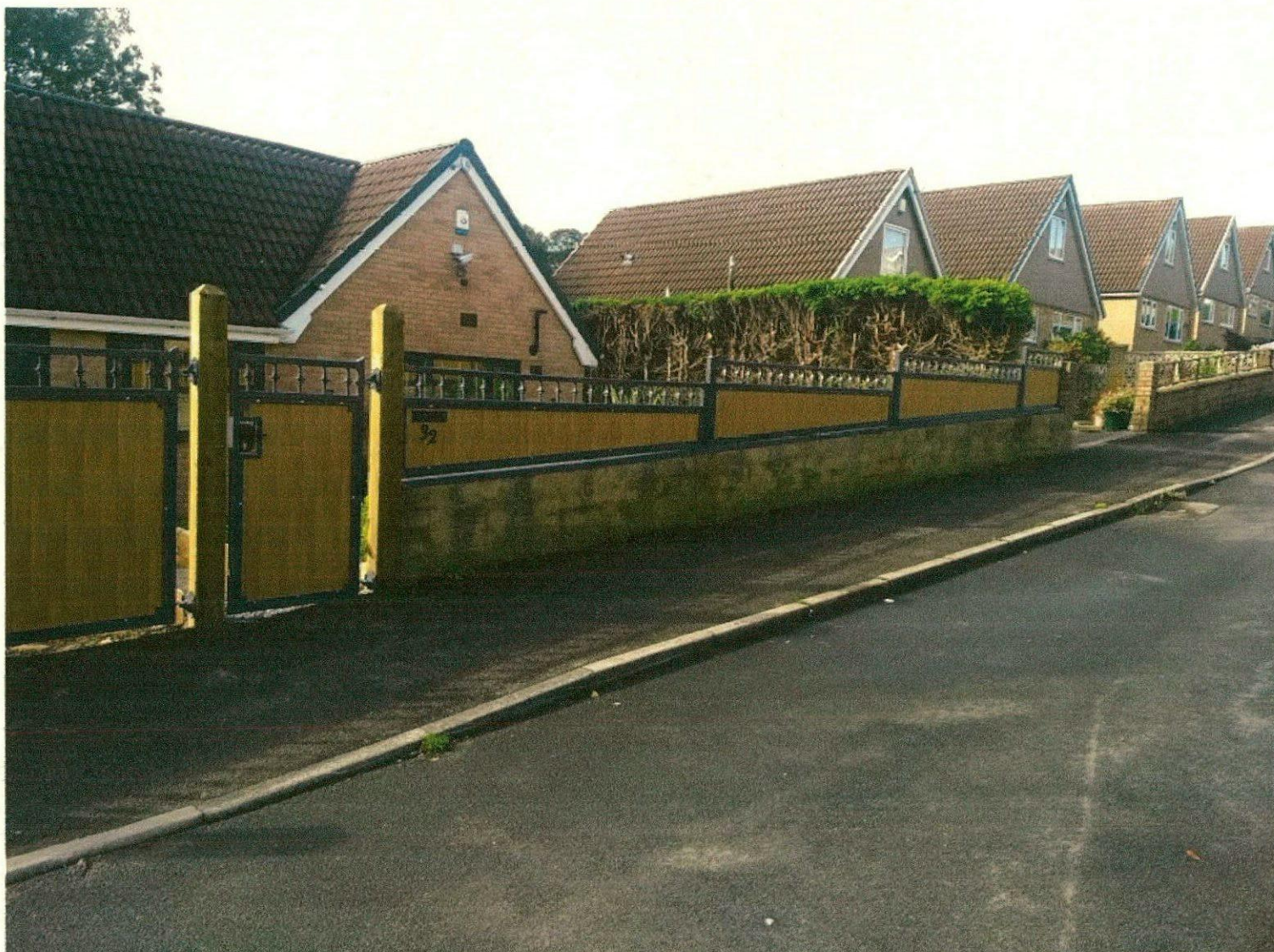
IMAGE 2 HONEYWELL PLACE SHOWING REPLACEMENT FABRICATED STEEL FENCE (UPPER VIEW)
