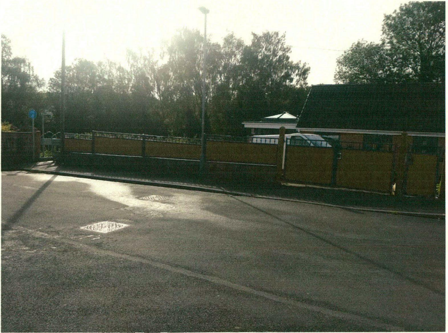
IMAGE 3 HONEYWELL PLACE SHOWING REPLACEMENT FABRICATED STEEL FENCE (LOWER VIEW)
