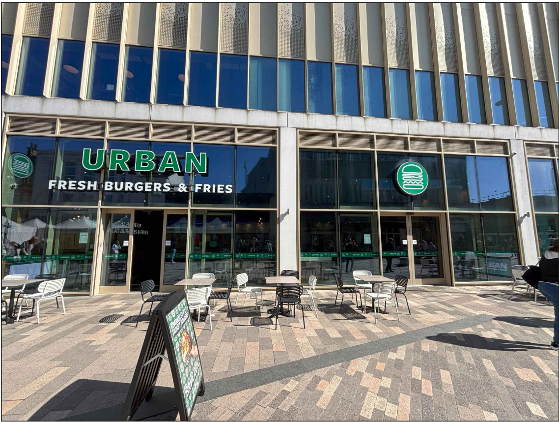
Existing Fascia NTS
