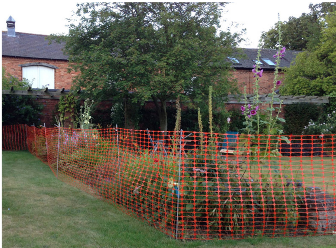
Figure 1: Plastic mesh fencing secured with heavy duty metal stakes
