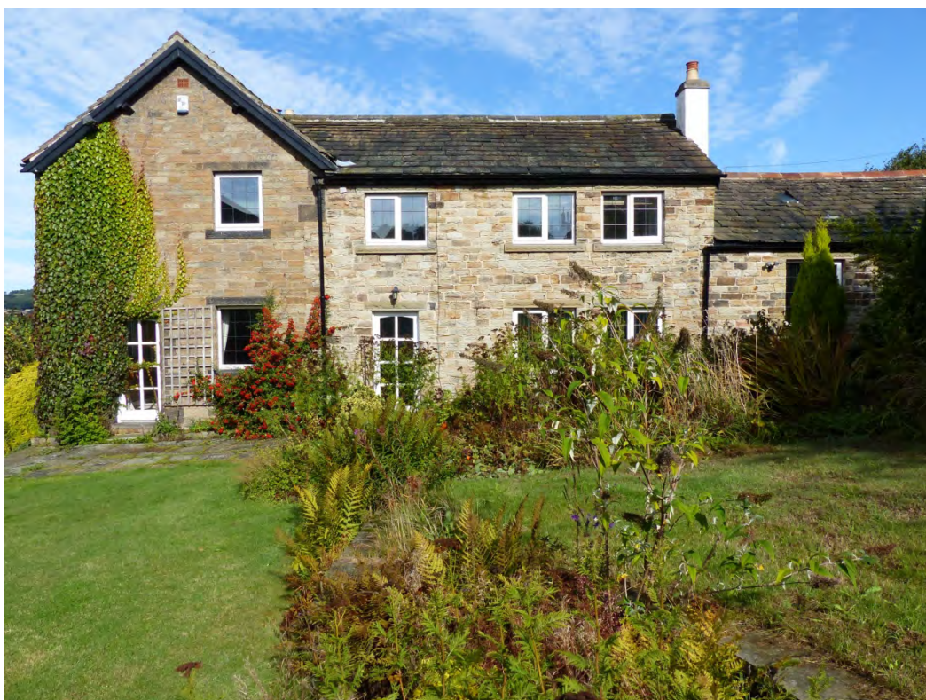
Plate 17: South elevation of 2 Hill Top, looking north
