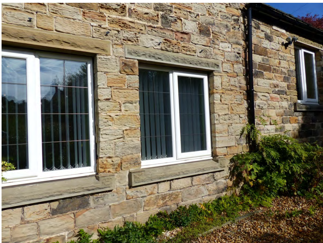
Plate 19: Detail of windows to central south elevation, looking northeast
