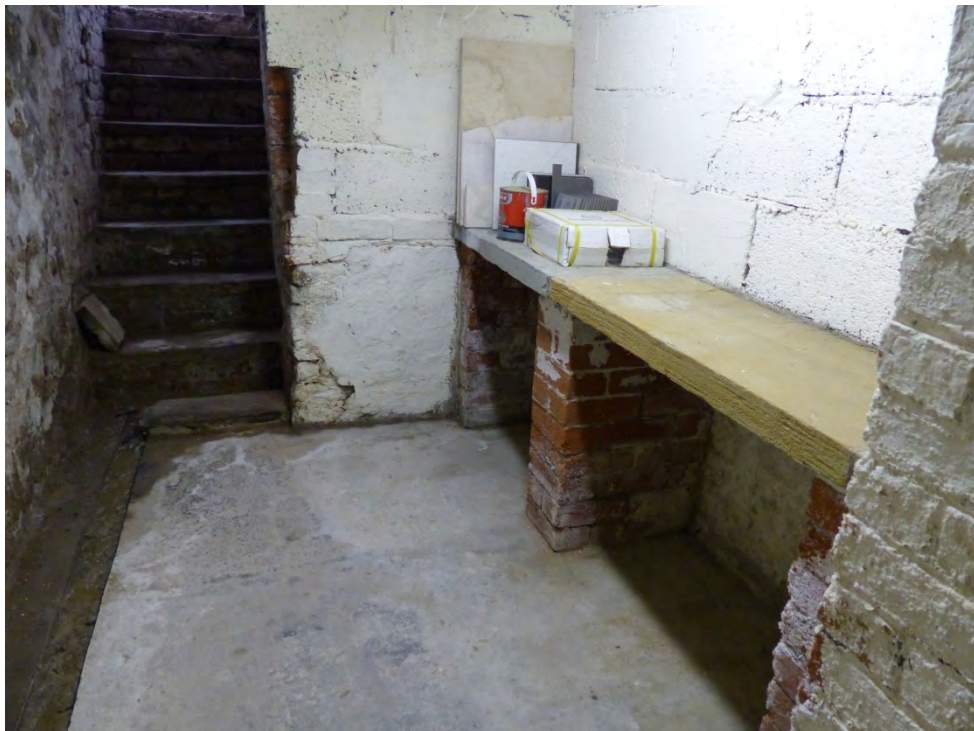
Plate 36: Stone benches in basement, looking east
