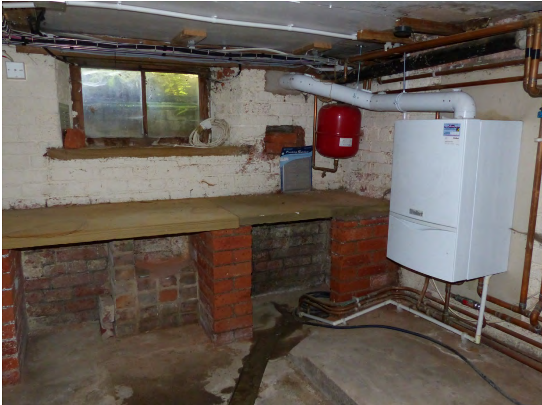
Plate 37: West end of basement, looking west
