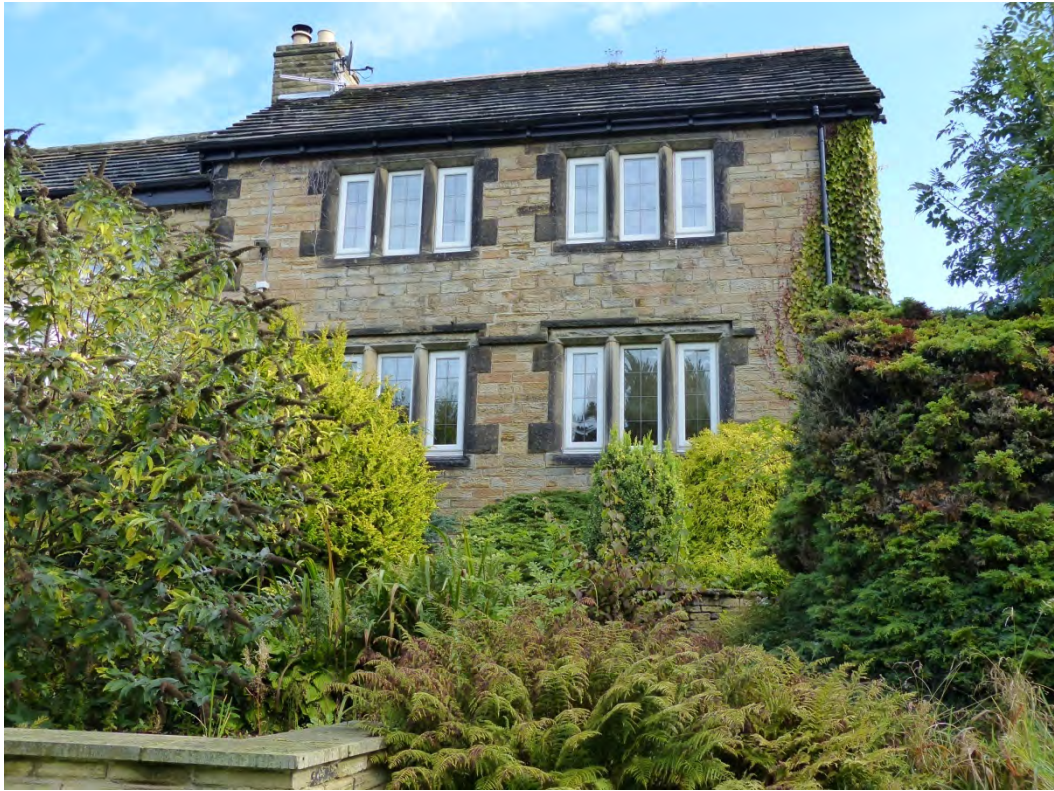
Plate 21: West elevation of southwest addition, looking east
