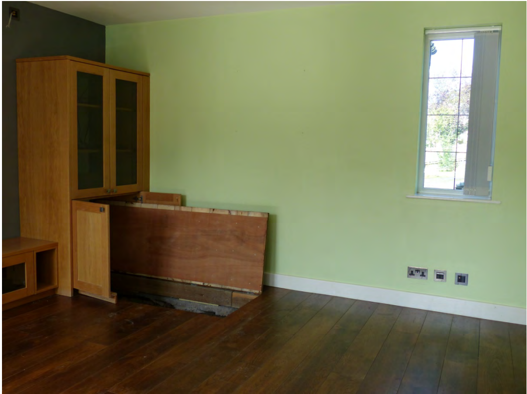
Plate 31: Living room in oldest part of the house, looking towards basement steps, looking northwest
