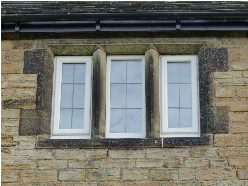
Plate 22: Detail of window to west elevation of southwest extension, looking east
