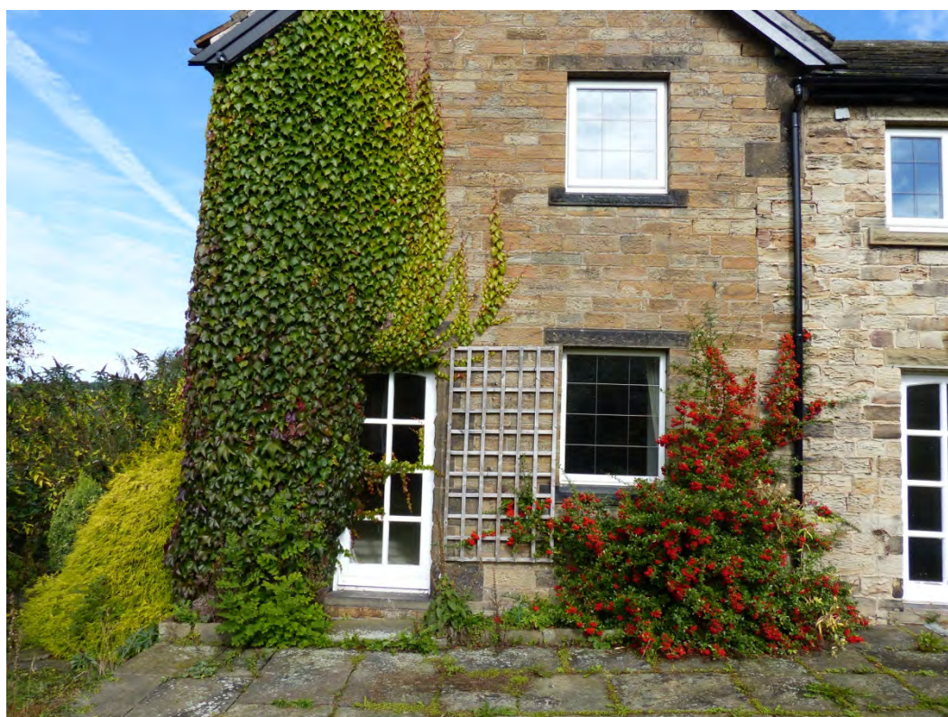
Plate 18: West end of south elevation, looking north
