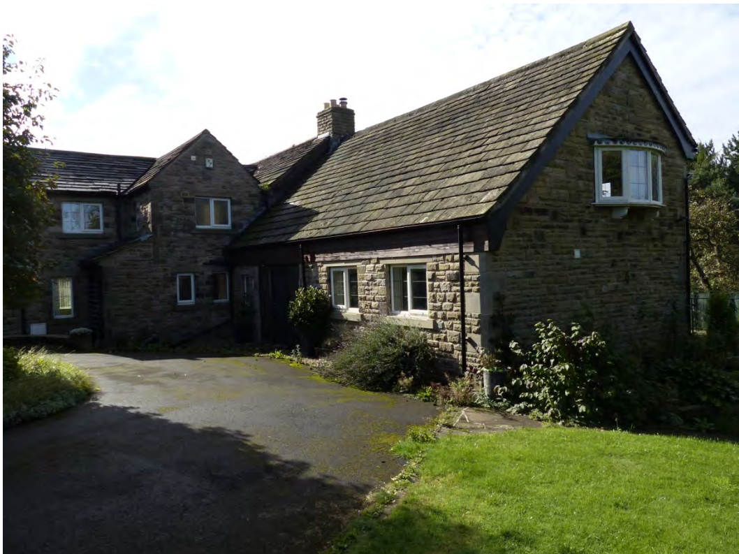
Plate 24: The northwest addition, looking southwest
