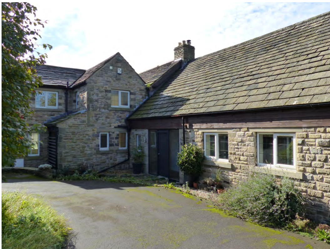
Plate 25: The east and north elevations of the house, looking southwest
