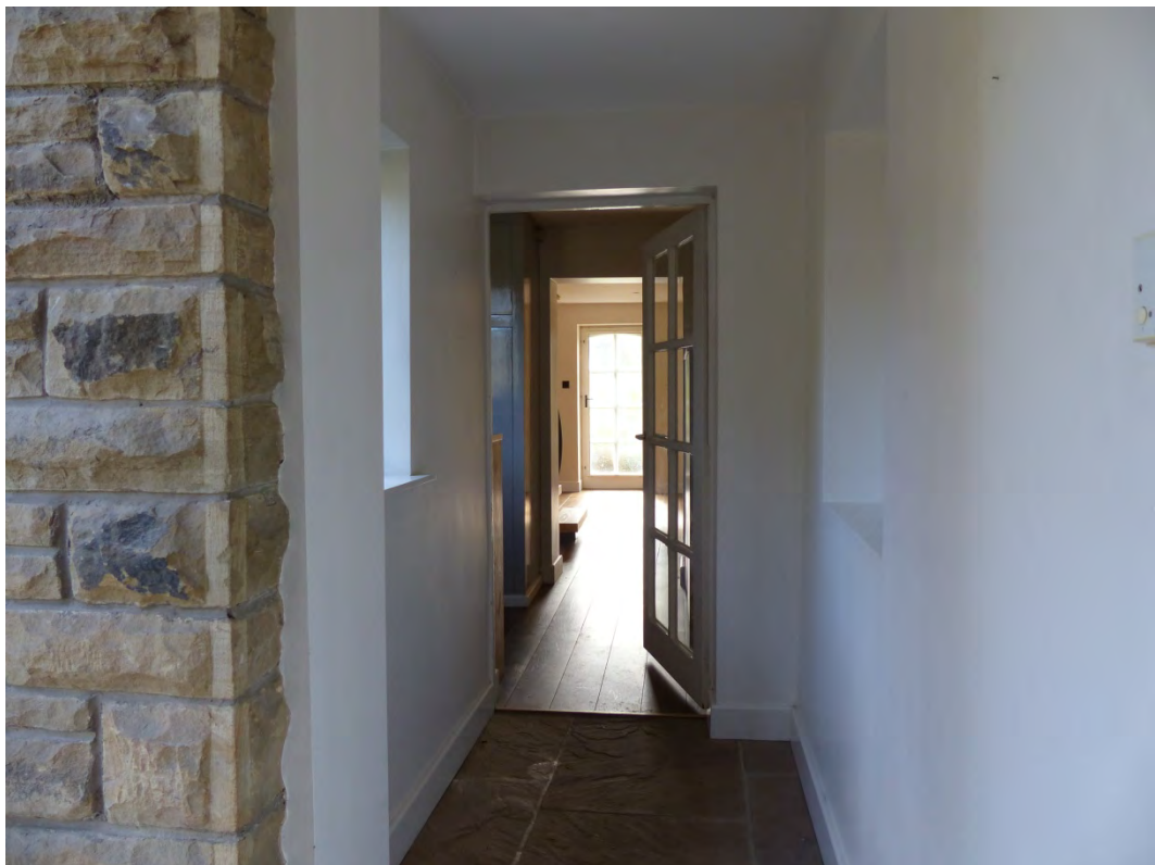
Plate 28: Hallway in northwest addition, looking south
