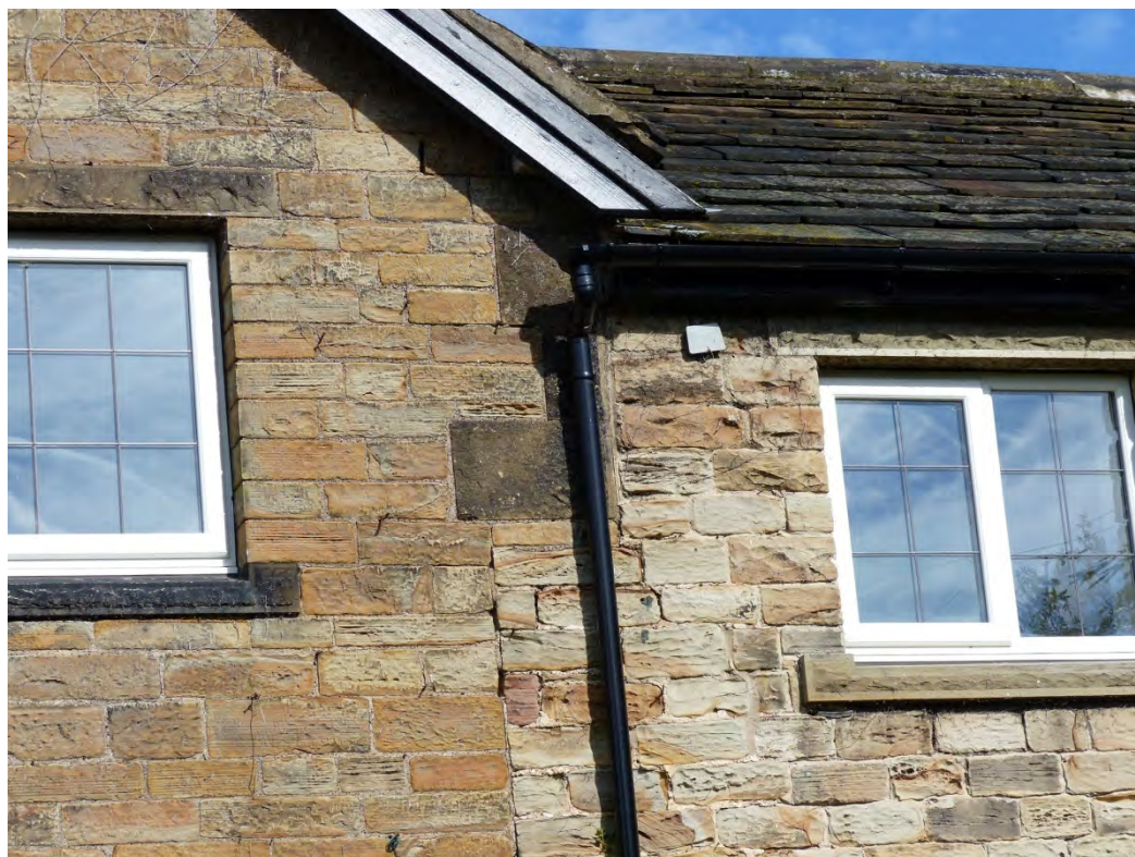
Plate 20: Junction of central elevation and southwest addition, looking north
