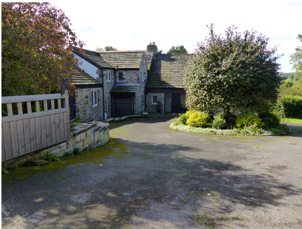
Plate 13: North and east elevations of the house as seen from the road, looking west
