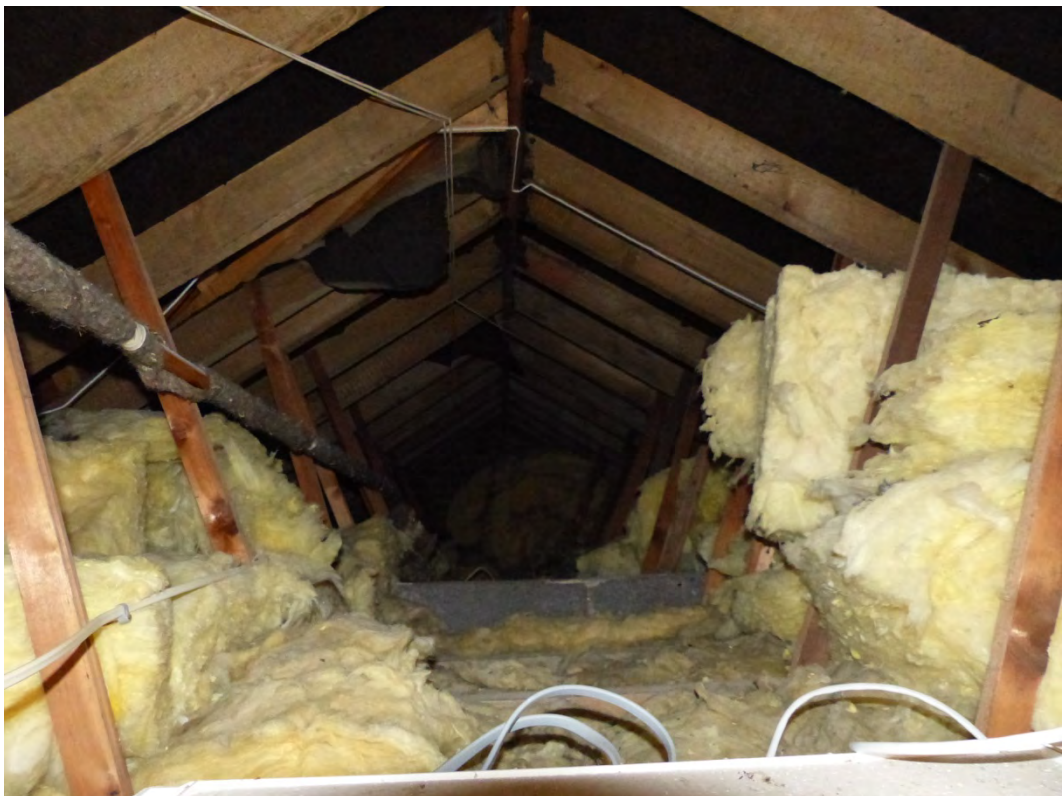
Plate 40: The internal roof above oldest part of the house, looking east
