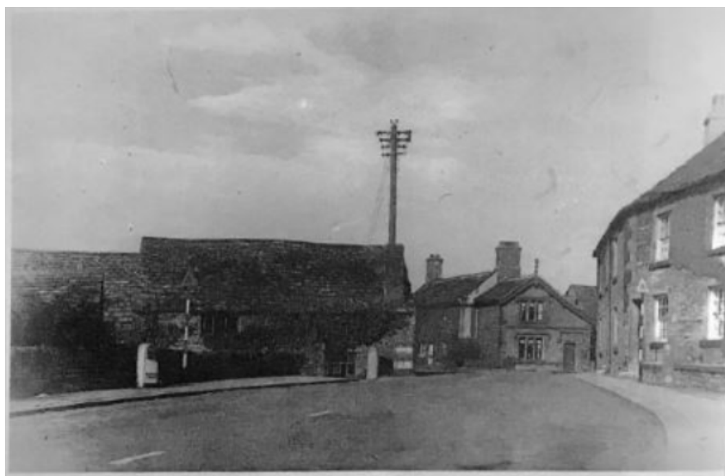
Plate 5: 1950s photo of Cawthornes first school and priest house, demolished 1962.
