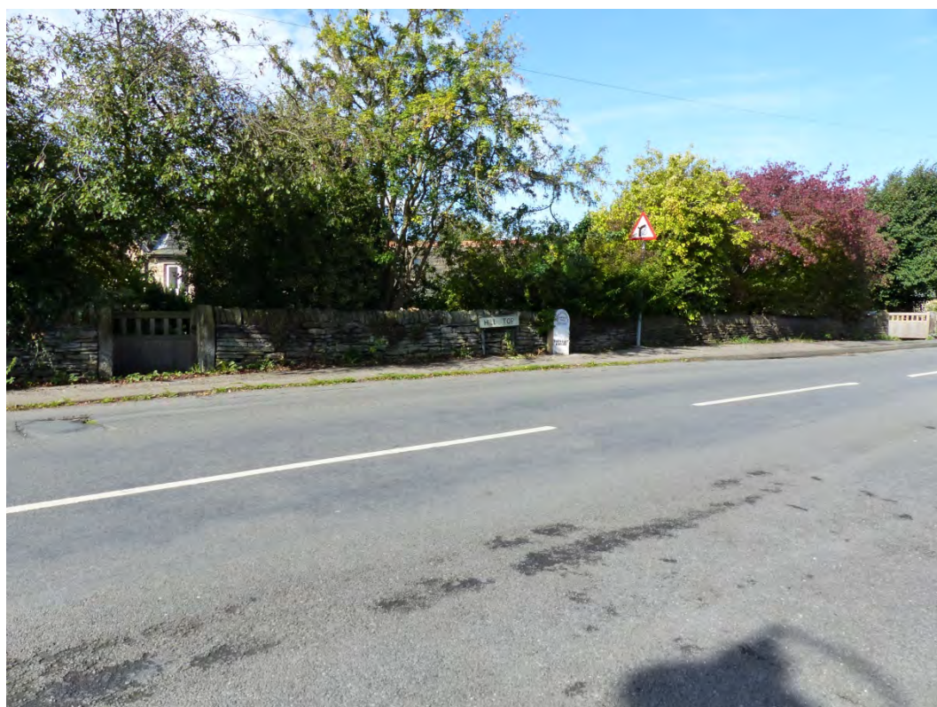
Plate 12: View of the milepost and boundary wall to the east of the house, looking northwest
