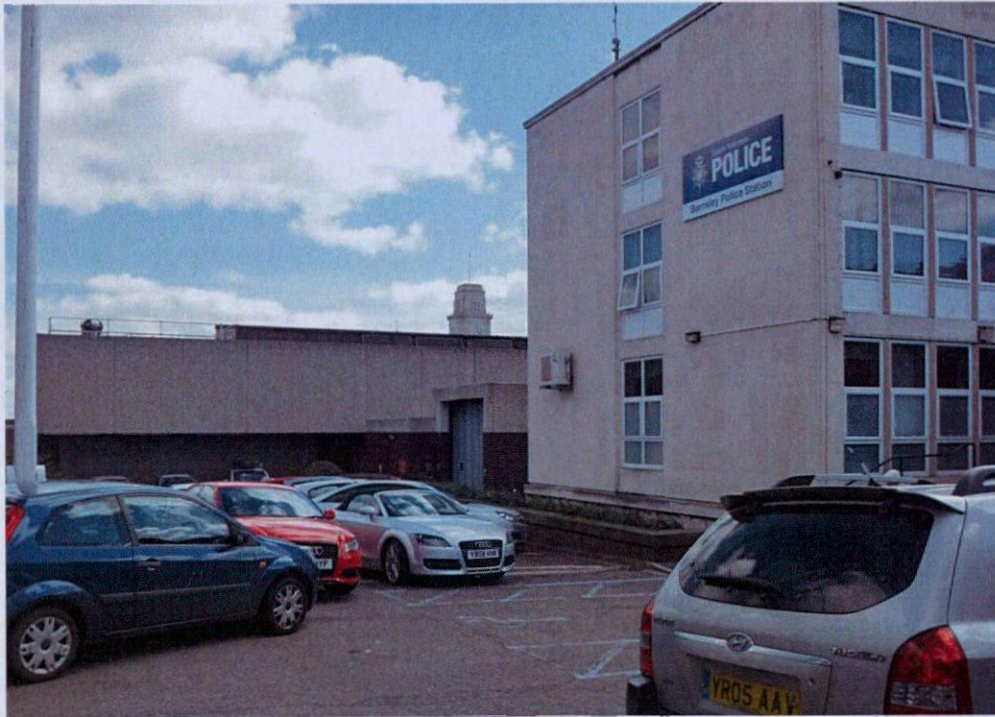
Plate 9: Three-storey block on site of North Pavement and National Spiritualist Church
